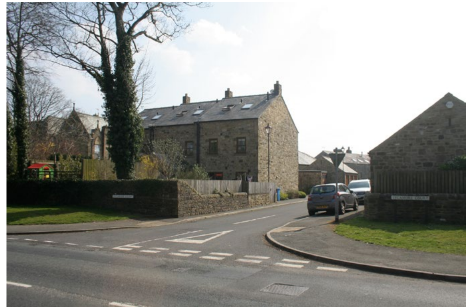
Development in the grounds of Thornton Hall
