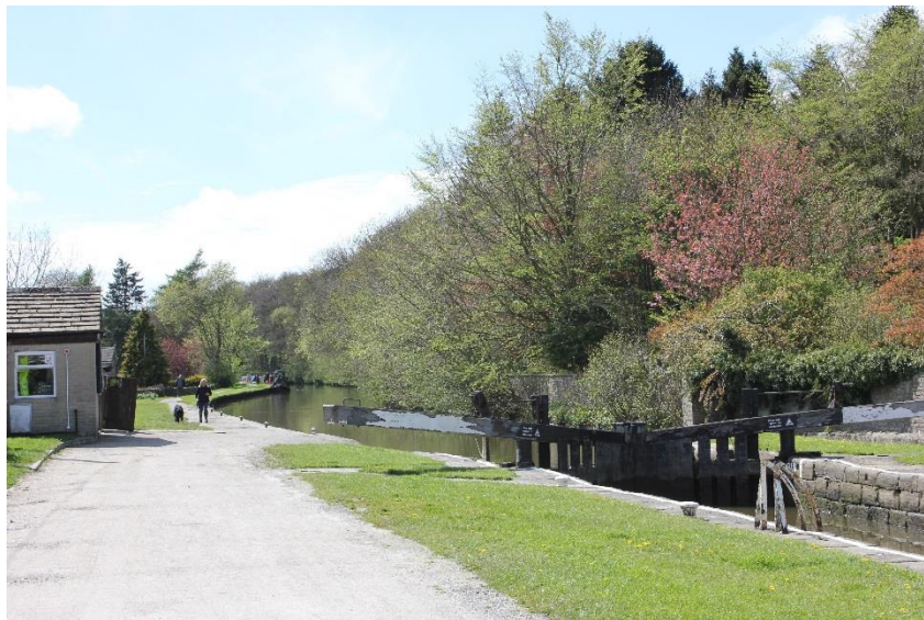
Higherlands Lock, Leeds Liverpool Canal
