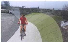
Regrade slope as much as possible to improve gradient, vehicle gate could be relocated to right of pedestrian gate giving more space for regrading of slope.
