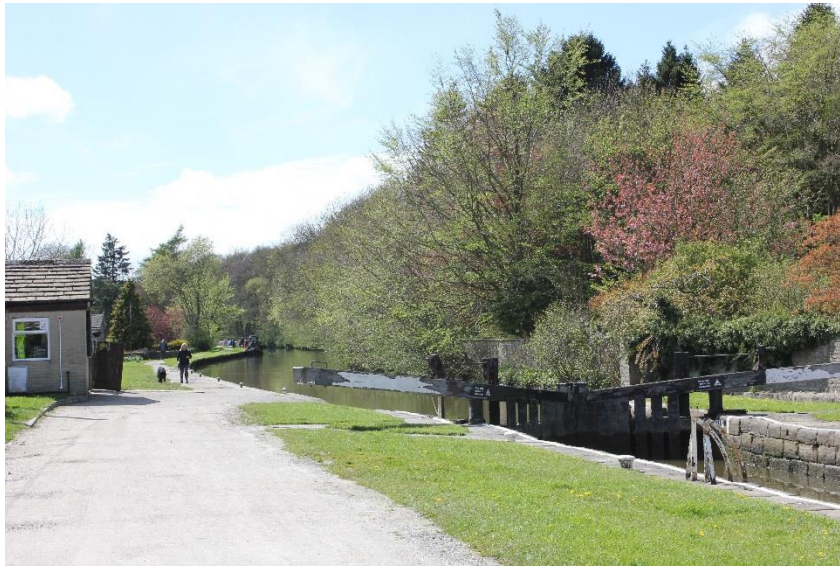
Higherlands Lock, Leeds Liverpool Canal
