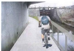
As towpath goes under A65 it sweeps left up steps next to the lock wall.
