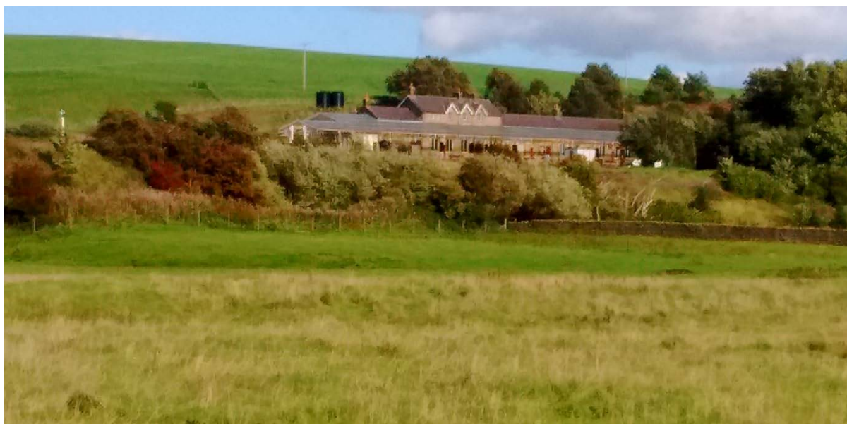
Fig 3 Significant degree of inter-visibility between Hellifield Station and the application site
