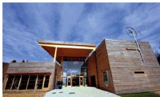
Figure 38 Building mounted wind turbine at Dalby Visitor centre in Ryedale (Source: Green design at Dalby visitor centre case study, Forestry Commission, 2010)
