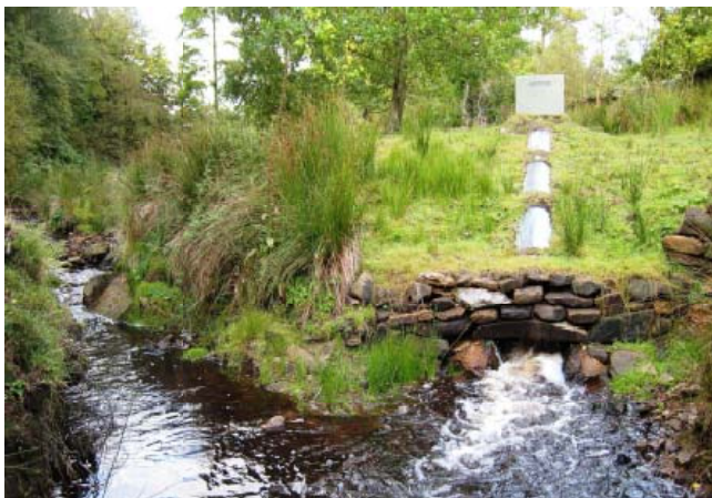
Figure 24 Bonfield Ghyll hydro facility in the North York Moors National Park (Source: Case study, Mann Power Consulting Ltd)
