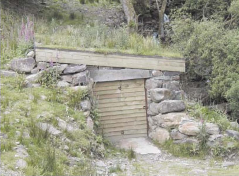
Turbine house for a 100kW hydro plant. Taken from Planning for Renewable Energy: A Companion Guide to PPS22 (OPDM), 2004
