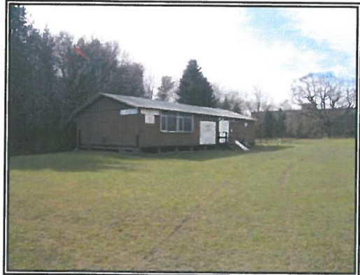
Photograph 5.8 Risedale High School pitch- side facility (IPF02)
