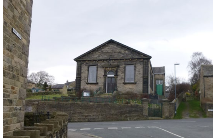
Methodist Church, Skipton Road
