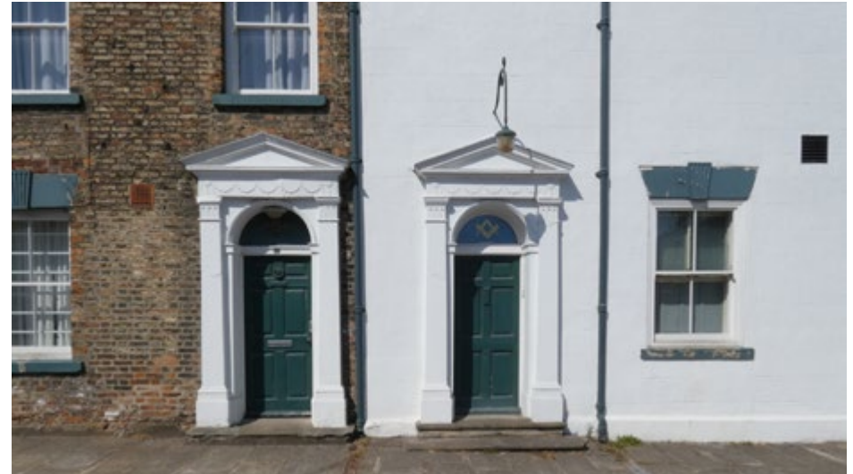
2.14 Late-18 th century doorcases with pedimented architraves and fanlights on Church Hill (Inshall)
