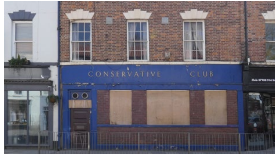
2.15 Late-18 th century sashes with exaggerated keystones and brickwork in Flemish bond (Inshall)
