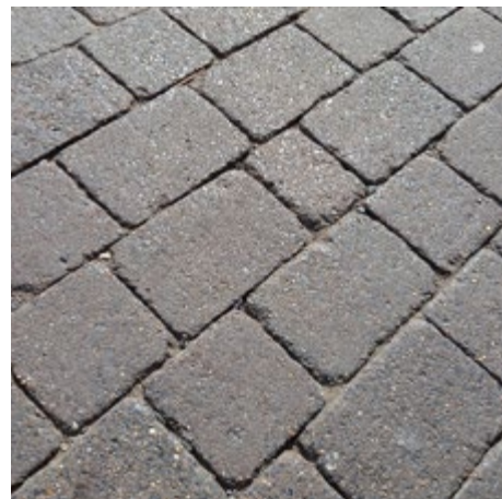
6.6 Textured concrete setts provide a suitable alternative to granite
