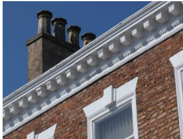
4.4 Well-maintained timber eaves cornice (Insall)
