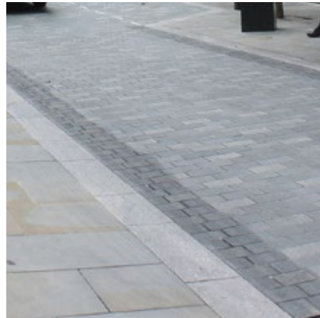
6.2 Flush kerbs help promote the sense of a 'shared space' on Bourdon Place, London
