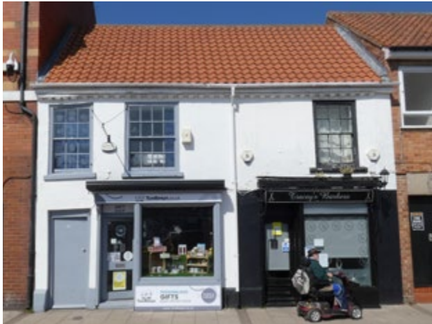
3.3 Mid-Victorian shopfront retaining awning fixings (Insal)
