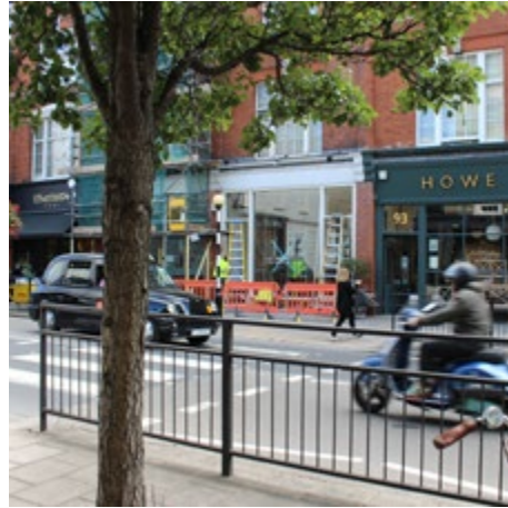
6.18 Guard rails should be black finish. Pimlico Road
