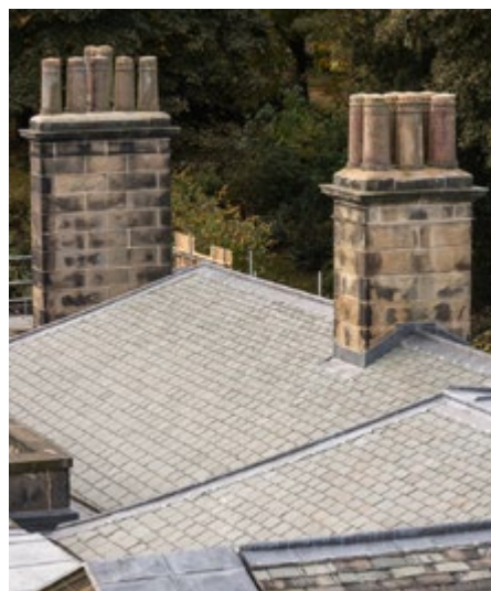
5.2 Newly laid natural slate roof (Insalls).
