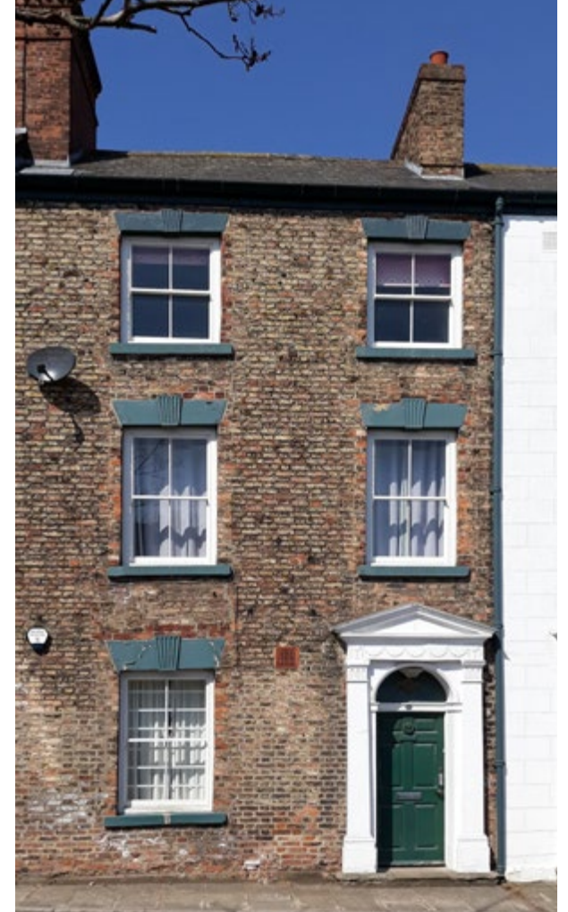
4.5 Colour-matched and neatly-arranged rainwater goods (Insall)
