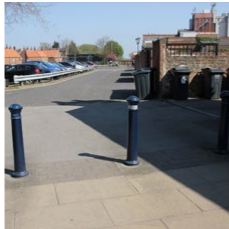
6.30 Avoid bollards in colours other than black, rear of Micklegate car park
