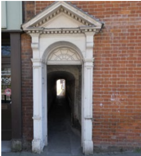
2.19 Georgian doorcase to alley at Park House, with pedimented architrave and overpainted fanlight (Insall)
