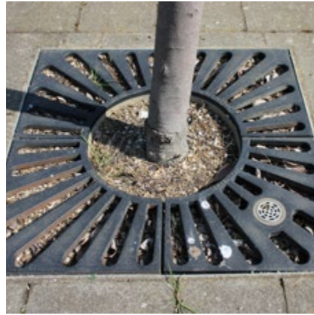
6.34 Tree grille finished in matt black, with aperture for fixing the inlet of an aeration/irrigation system on Riverside Gardens
