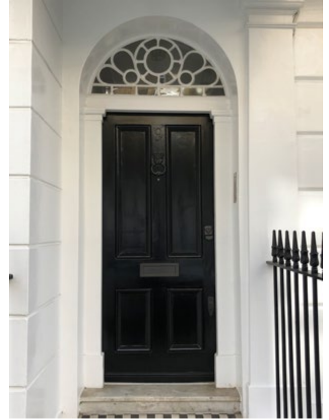
4.11 Refurbished Victorian door and fanlight (Inalls)
