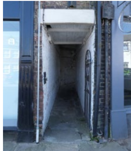
2.20 Typical opening to alley with timber lined soffit and painted brick walls (Insall)
