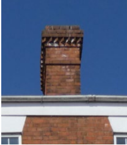
4.1 Brick chimneystack with decorative cornice, Micklegate (Insall)
