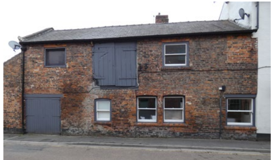
2.5 Small-scale industrial building (Insell)
