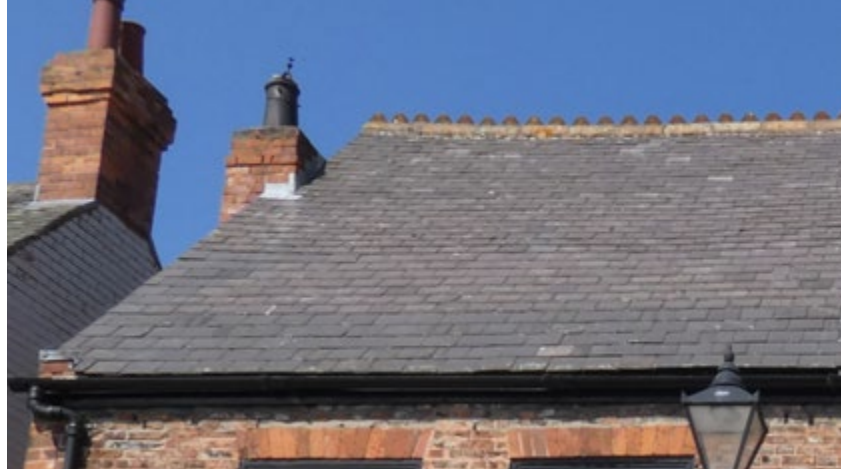
4.2 Slate roof with clay ridge tiles (Insall)
