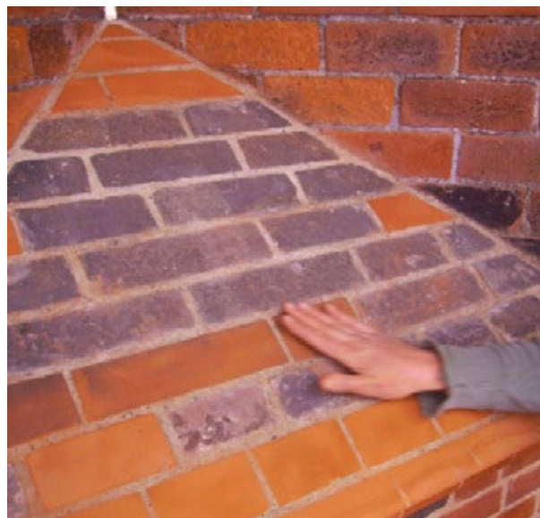
4.7 Repointed chimneystack (Install)
