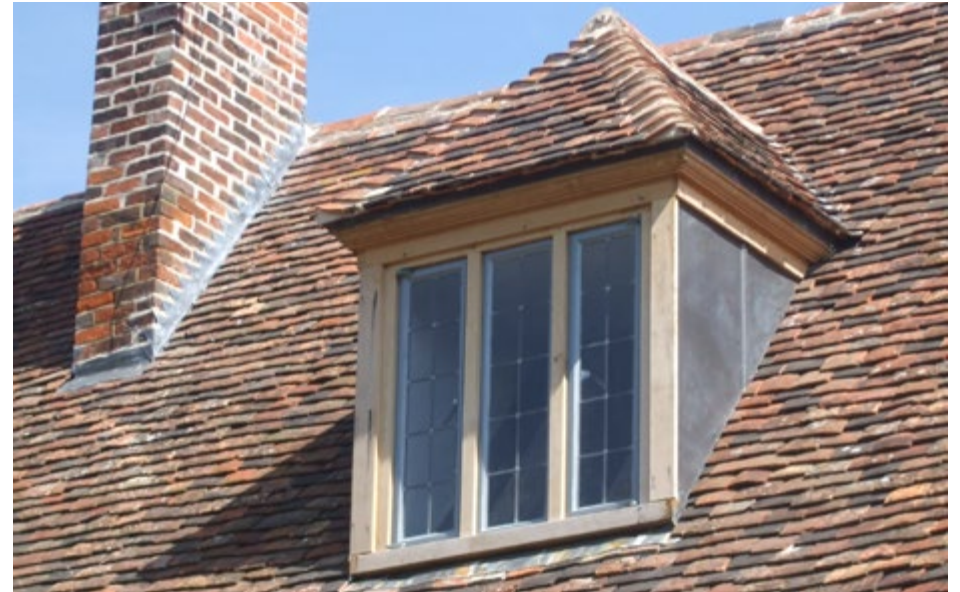
5.6 New dormers on a medieval property in Sittingbourne (Insalls).
