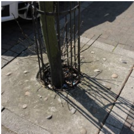
6.36 Avoid concrete inset to tree pits, on Micklegate
