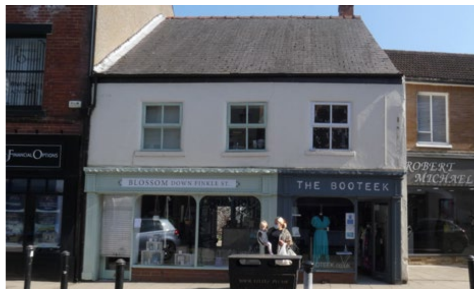
5.17 Soft tones and muted colours to the facade and shopfronts (Insall)
