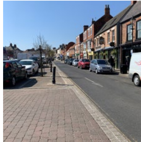
6.11 Concrete block paving on Micklegate
