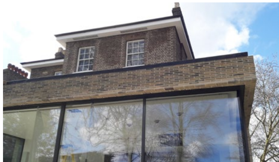
5.1 New extension with brick carefully matched to the historic main building (Insalls)
