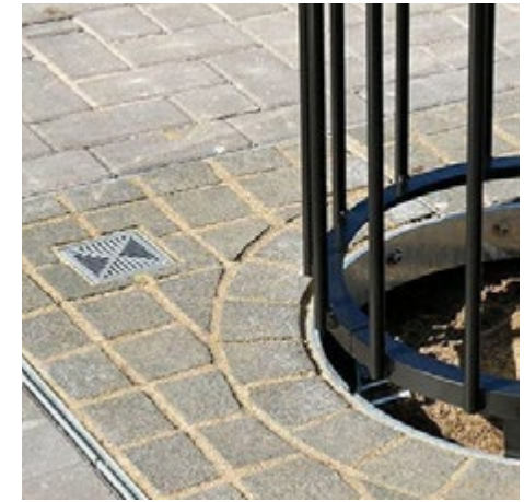
6.39 Tree grille inset neatly within surrounding paving (©GreenBlueUrban)
