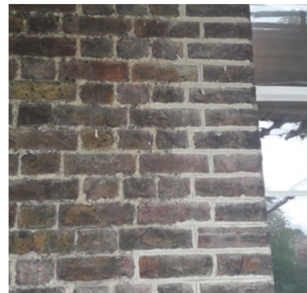
4.8 Repointed brickwork to corner (Install)
