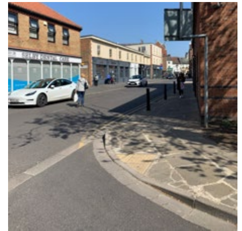
6.16 Avoid odd angles to tactile paving and excessive cuts (on New Lane)
