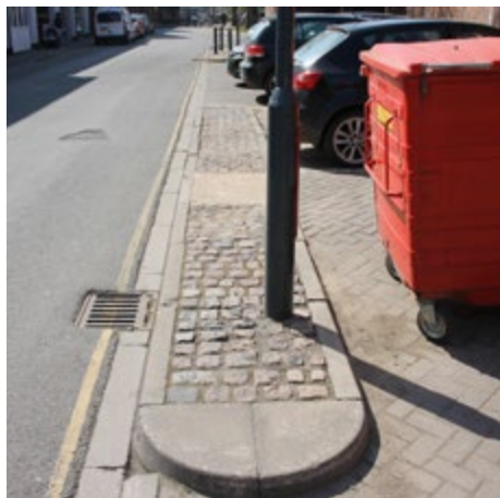
6.5 Channel edging to road surface with small unit setts used as fill, on James Street
