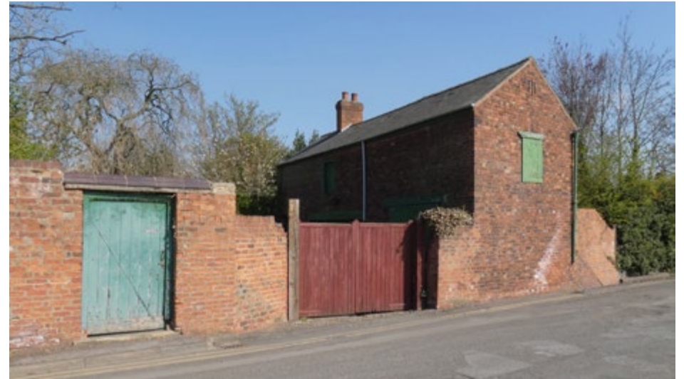
2.17 Simple plank and rail gates and doors in a backland area (Insall)
