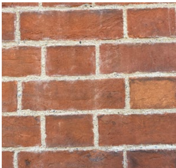
4.6 Lime mortar joints (Install)
