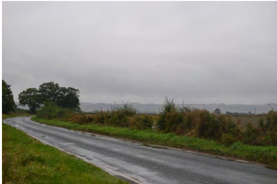
Rural roads cross the vale, delineated by grassy verges, which provide important green linear corridors
