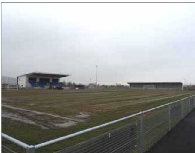
Ground from the northwest corner
