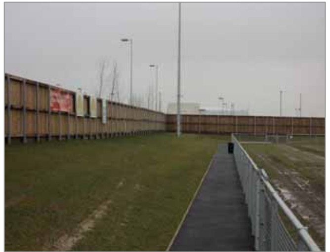
Open standing / land for future development
