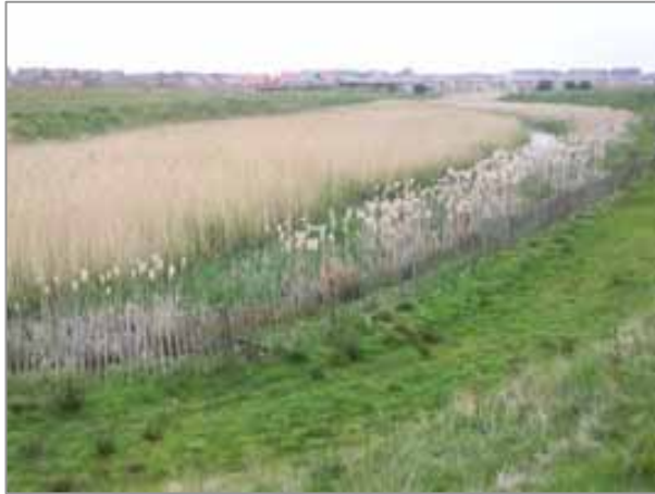
Image 6.9: Example of attenuation pond
