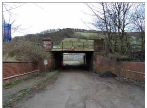
Image 3.8: Secondary access under height restricted railway bridge
