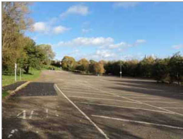
Image 3.9: Hard standing to the north of the site
