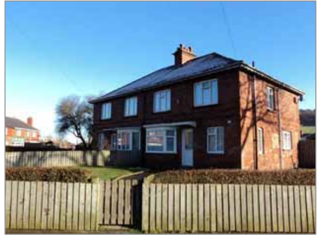
Image 22: Example of semi-detached housing close to the site
