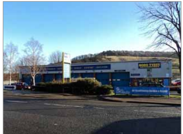
Image 32: Single storey retail warehouse along Seamer Road
