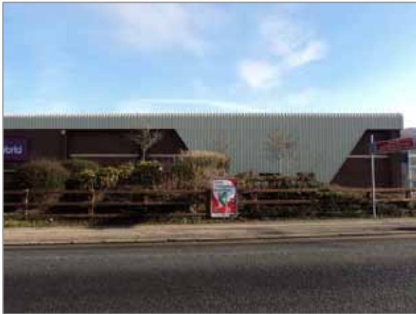
Image 29: 'Inactive' elevation of retail warehouse along Seamer Road
