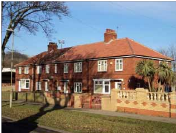
Image 23: Example of small residential terrace close to the site
