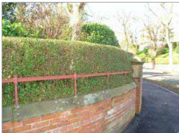
Image 6.1: Boundary wall with iron rail
