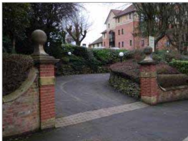
Image 6.2: Gate piers with stone cappings
