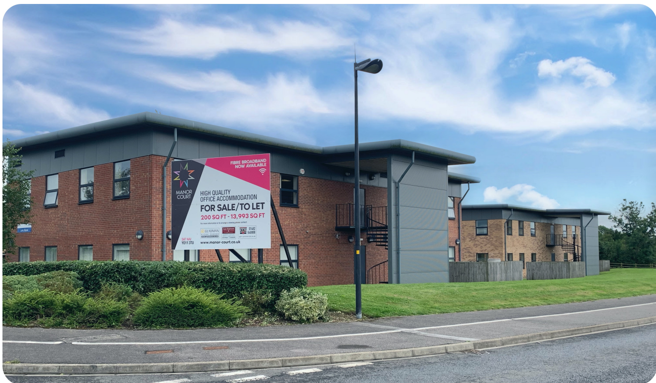
Picture 9.1 Offices at Scarborough Business Park
