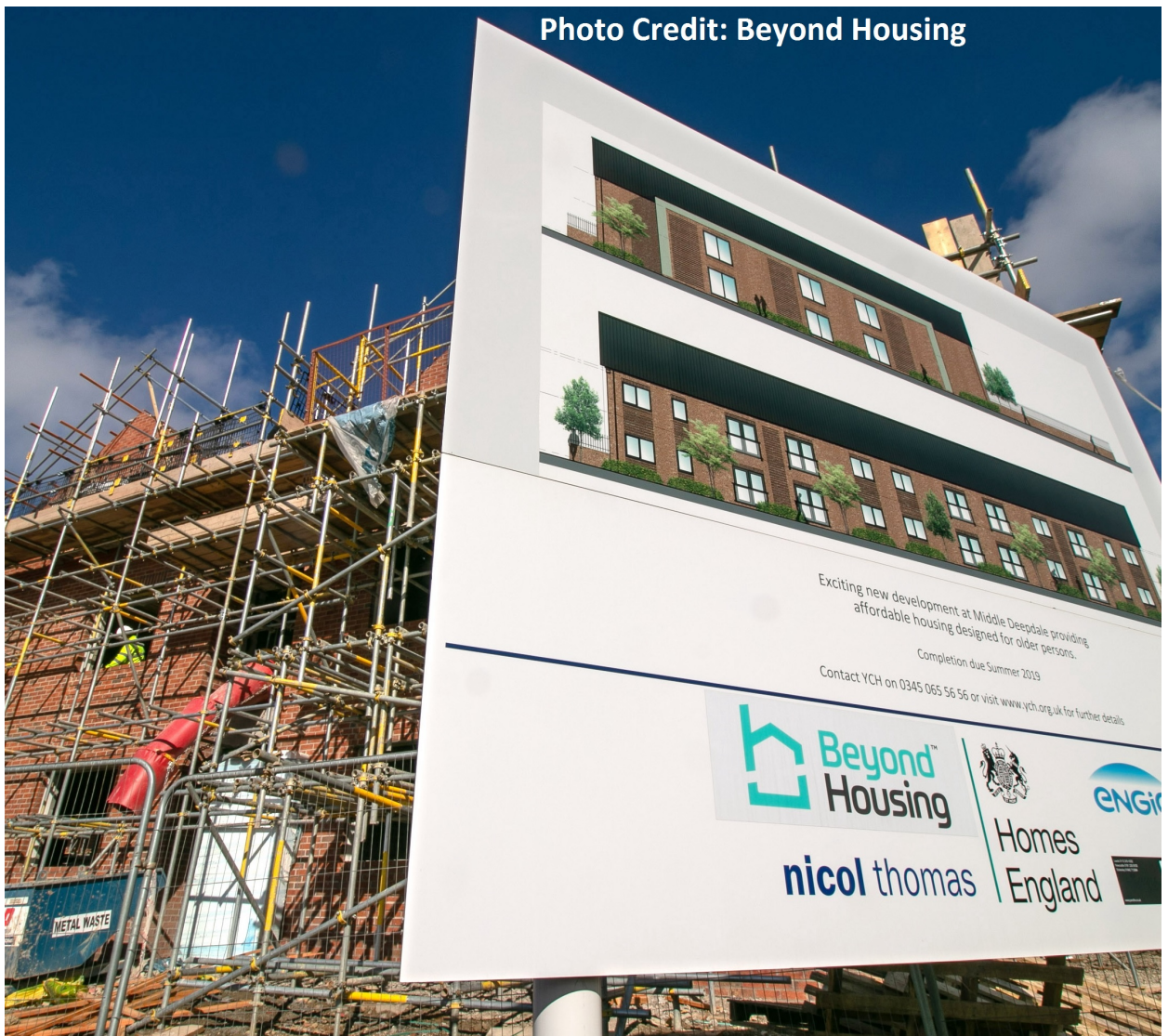
Picture 5.3 Affordable Homes Construction (Credit: Beyond Housing)
