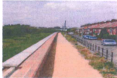
Brick-clad flood wall near Ousebank Cottages
