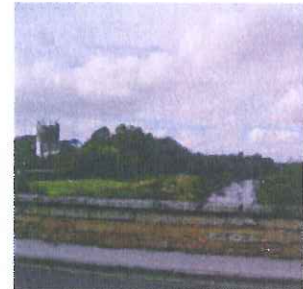
Flood defence banks in Tadcaster and Selby
