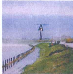
Selby's flood defences in the 2000 flood
