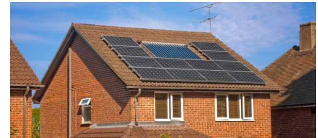
Right: Solar PV and Solar Thermal Panels (Credit: www.thegreenage.co.uk )
