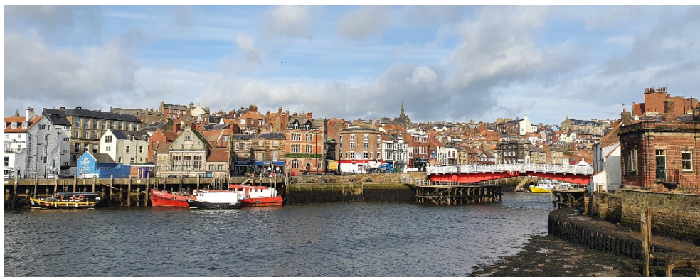
Figure 6.53: View of New Quay Road and of the Swing Bridge, from Church Street
