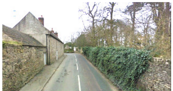
Buildings that abut the narrow footpath and high stone walls create a narrow “corridor” effect.
