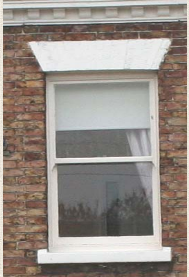
Above: white timber sliding sash Top left: Arch topped window Middle left: Variation on arch topped window Bottom left: Roof window in gable wall
