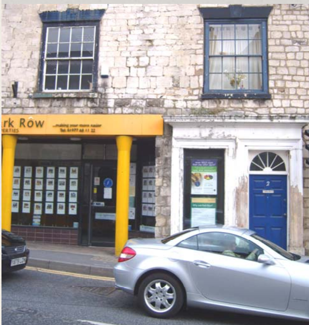
Right: The Fairways off Low Street. Above: traditional shop front in keeping with the building and modern unsympathetic alteration next to it.
