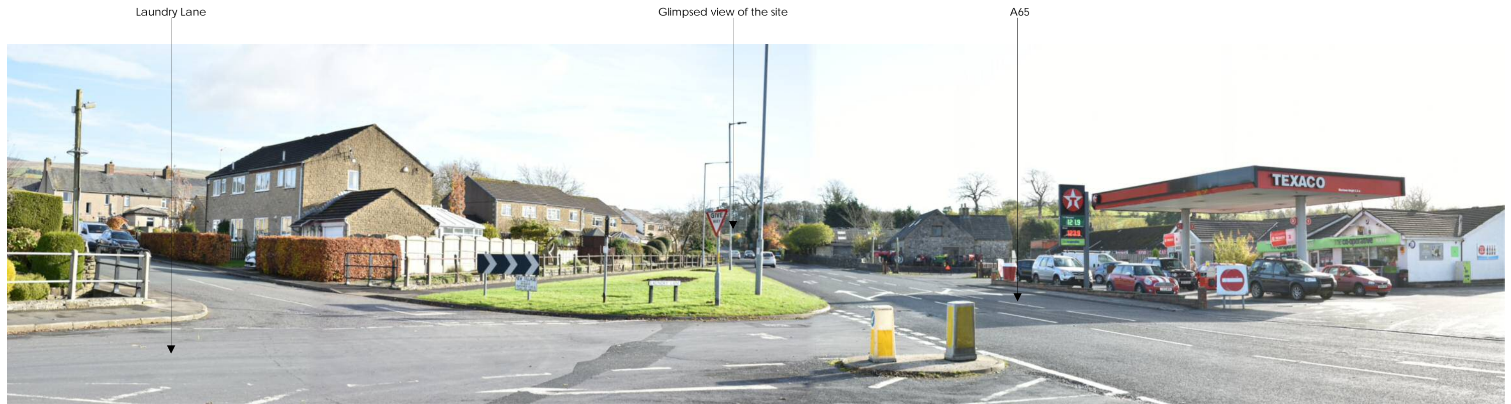
View 14 - From the A65 at the junction with Laundry Lane approximately 275m from the site looking east
