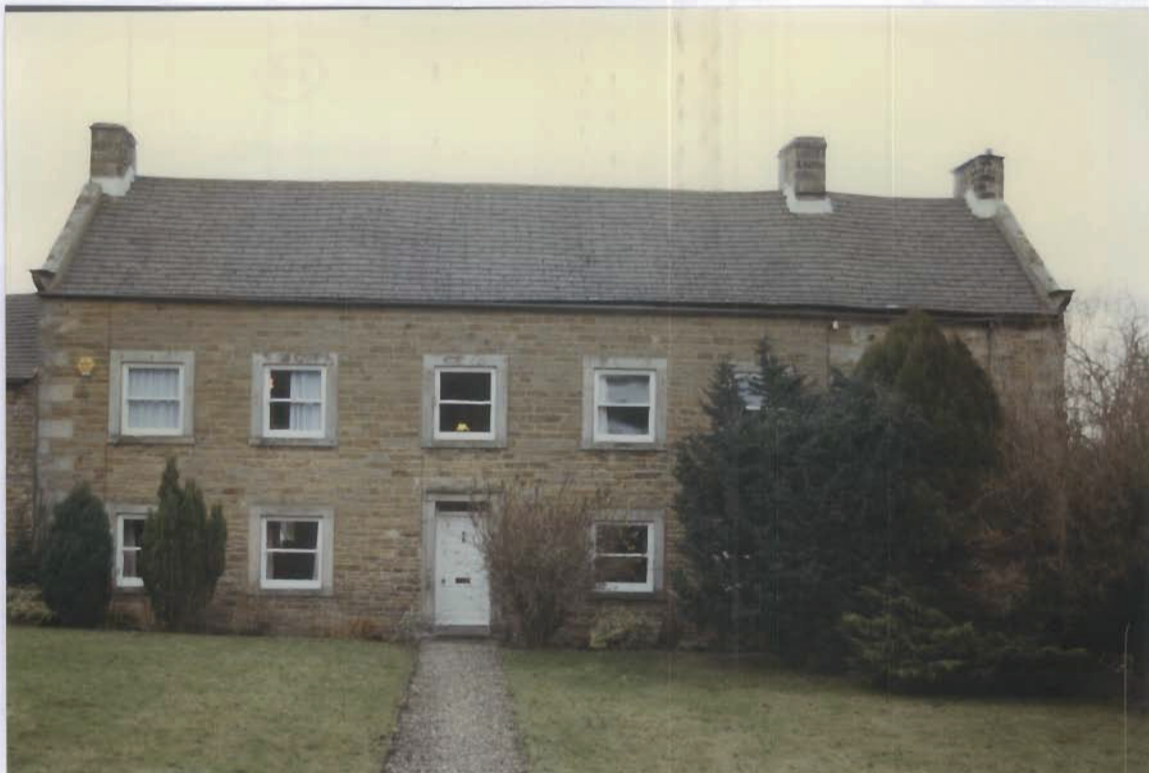
Whashton Lodge : the south elevation is built in high quality squared coursed rubble. Details of particular interest include flush quoins, shaped kneelers, stone copings and the dressed stone surrounds to the windows (which originally had flat faced mullions)
