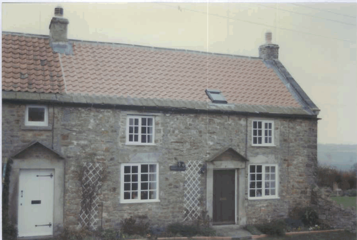
triangular slat4 hood or canopy above the heavy plain ashlar door surround at Cobblers Cottage
