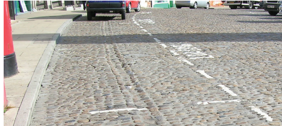
Figure 34: Original channel set into the historic cobble surface.
