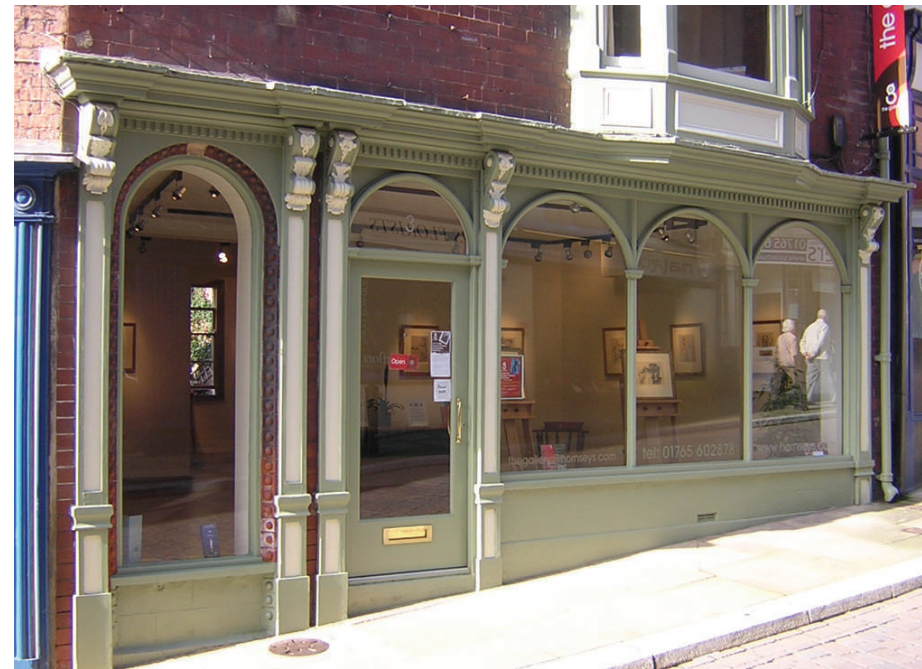
Figure 16: The successful application of heritage colours to a shopfront. The use of two colours is successful, but any more would be garish.
