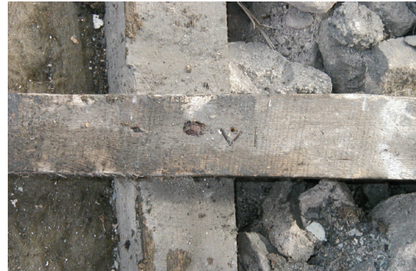
Figure 26: Carpenters marks and other historic details should be saved.
