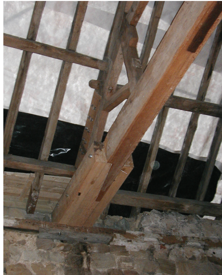
Figure 27: Traditional splice repair to tie beam.
