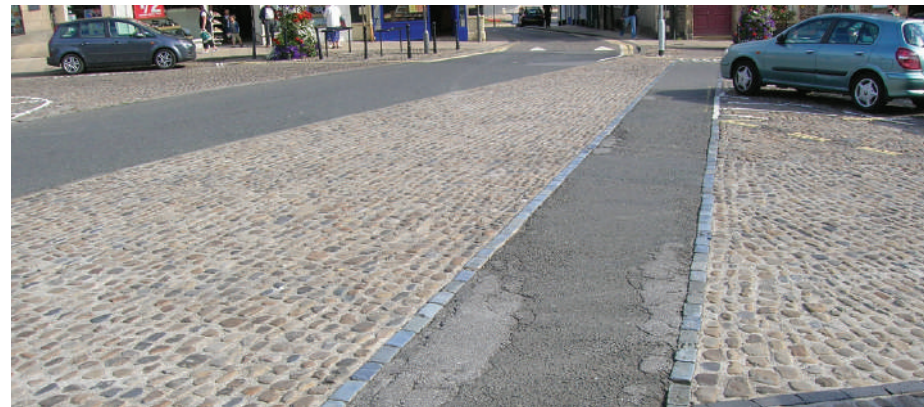
Figure 35: Poor use of modern materials detracts from the appearance of the historic streetscape.
