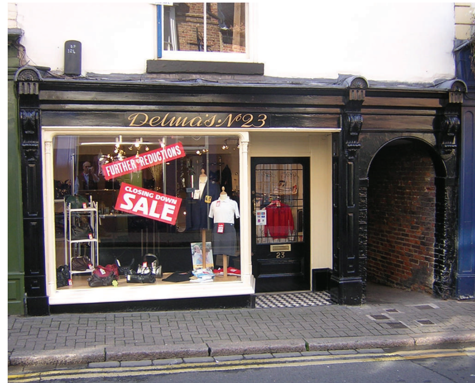
Figure 14: Late Victorian shopfront with heavily detailed pilasters and deep cornice (incorporating lead covering).
