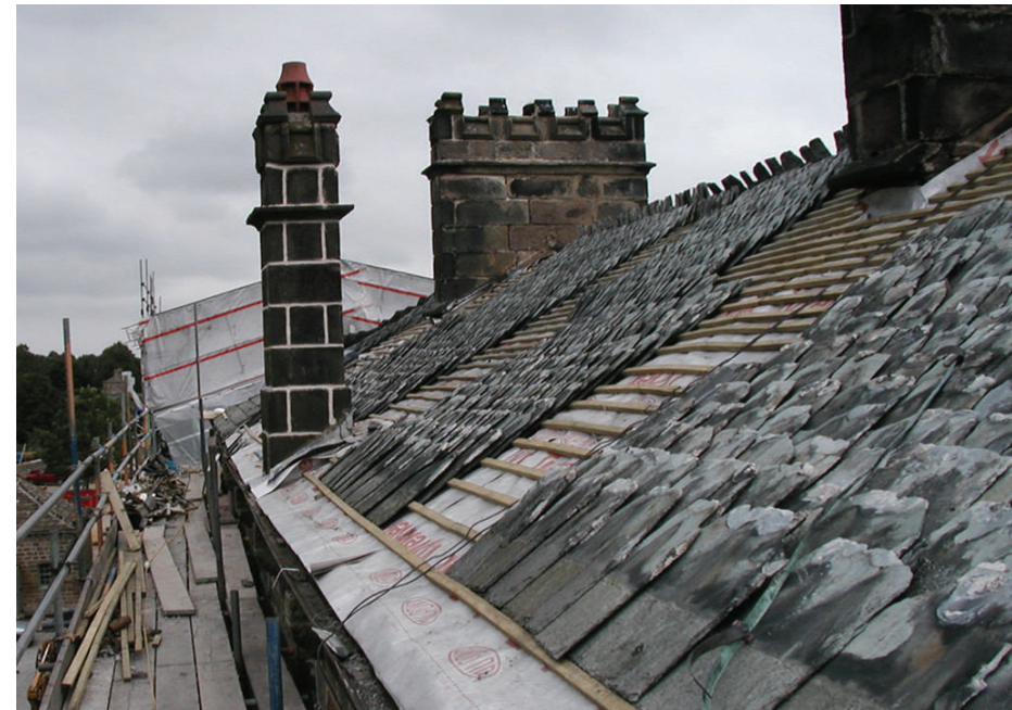
Figure 21: Slates stacked in diminishing size ready for laying
