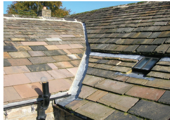
Figure 20: A well maintained stone slate roof.
