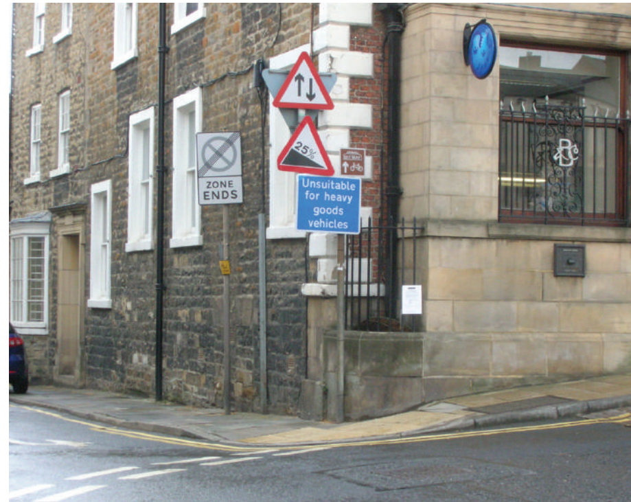
Figure 38: Over provision and poor siting of traffic signs.
