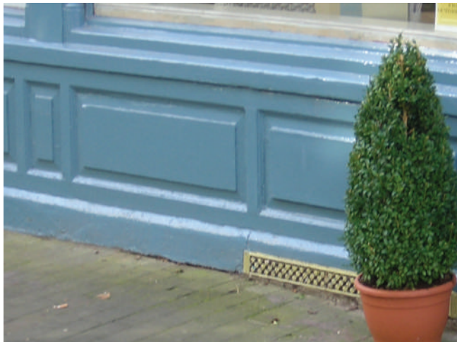
Figure 15: Stallriser from early Victorian style shopfront.
