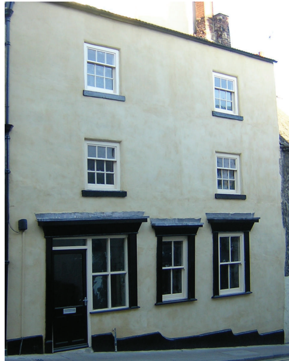
Figure 30: Traditional lime wash applied to lime render (note Figure 25)
