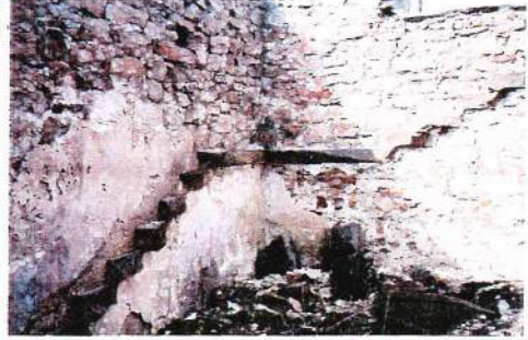
Figure 11. The Grandstand: staircase hall
