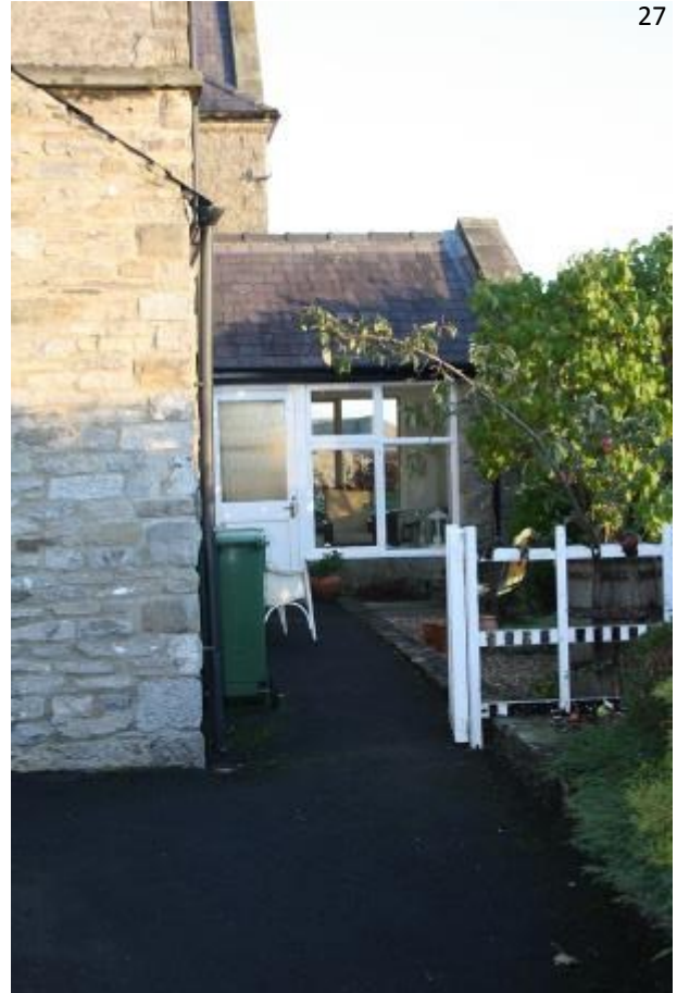
This is off-set to the left with a tripartite feature window filling the rest of this element. Two large porches provide access to each wing of the building. (photo 27)
