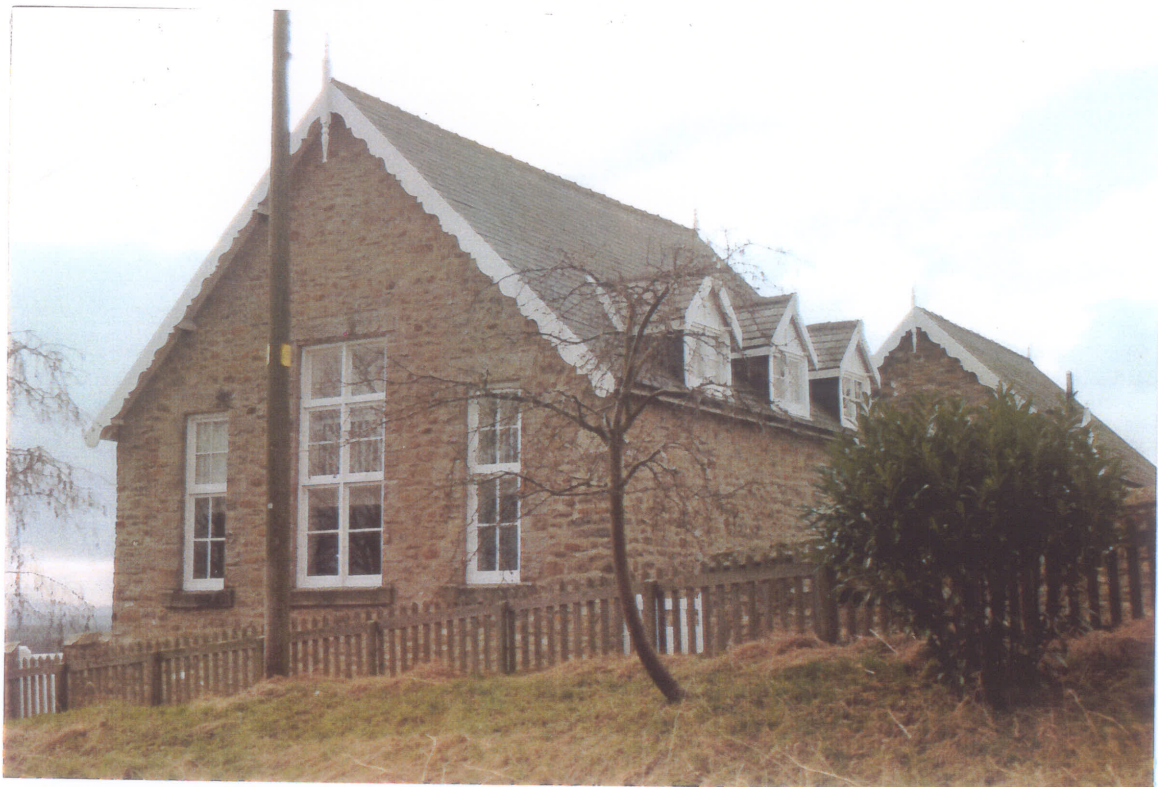
former School, now converted to a dwelling
