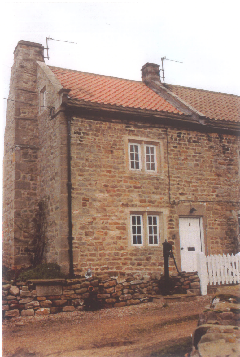
1 Pump Street, which dates from the mid-late C17, displays an array of interesting architectural features, including double-chamfered mullion windows, dressed quoins, kneelers and water tabling
