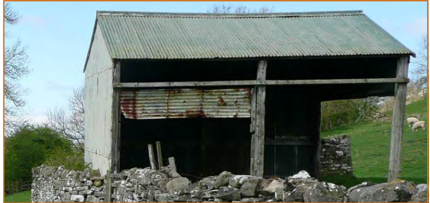
Figure 31: Timber-framed shed with corrugated cladding to north of village (photo © Gaby Rose, YDNPA, 2017)
