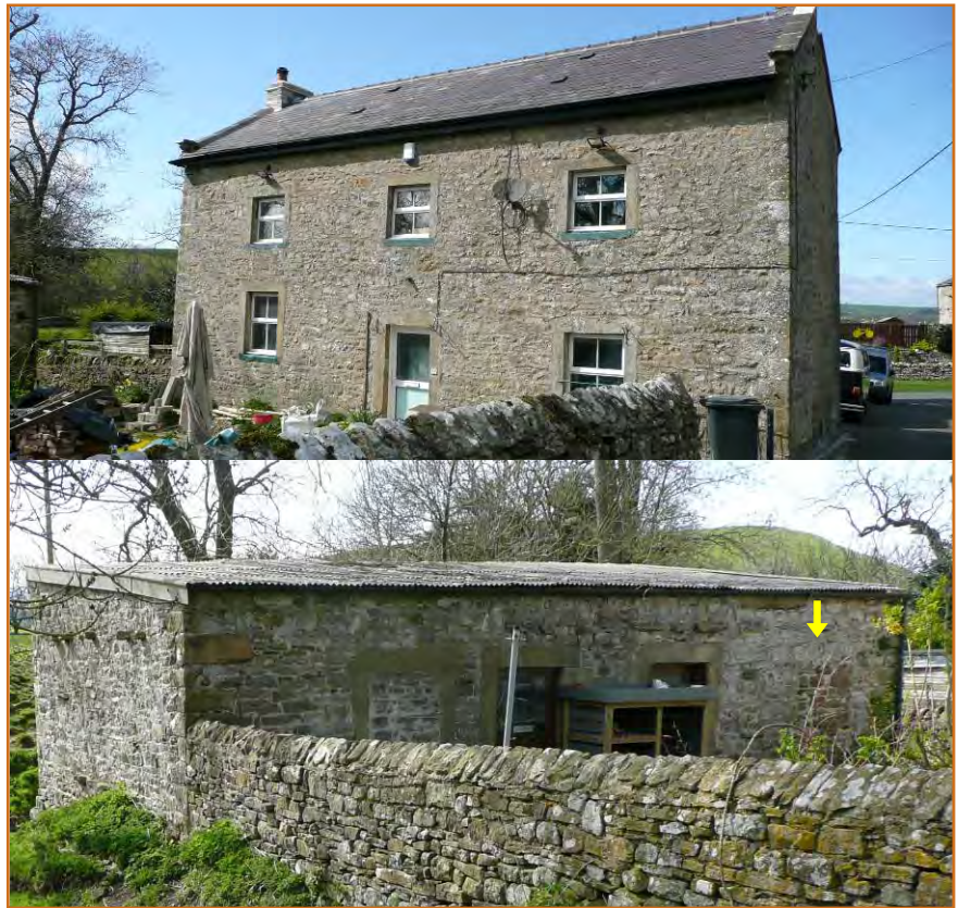
Figure 39: No. 10 and curtilage outbuilding to the left/southwest; note the imported roof slates to the house; the arrow shows the location of the later, now blocked flat-arched opening (photos © Gaby Rose, YDNPA, 2017)
