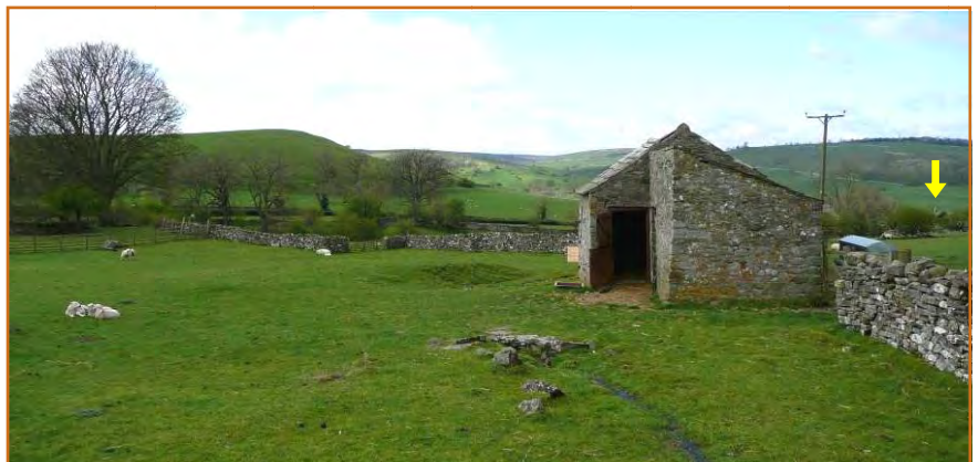
Figure 20: View 7, field barn with How Hill on the left in the background and the arrow on the right pointing to the church; note the line of telegraph poles (photo © Gaby Rose, YDNPA, 2017)
