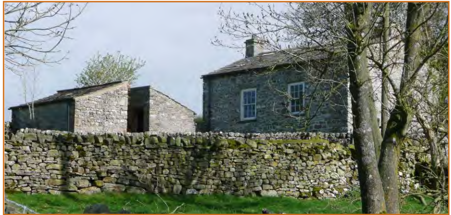
Figure 41: Former school with flat-arched windows and two small mono-pitched outbuildings (photo © Gaby Rose, YDNPA, 2017)
