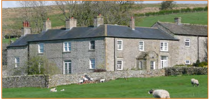
Figure 40: Manor House, with some flat-arched window openings; note the elaborate entrance porch (photo © Gaby Rose, YDNPA, 2017)
