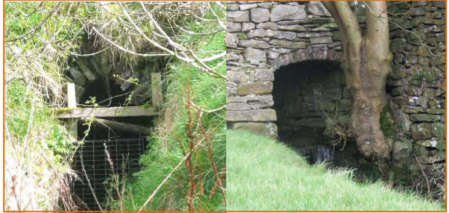
Figure 44: Features of local interest: Left: culvert at level opposite North House (photo © Gaby Rose, YDNPA, 2017); Right: culvert behind converted barn and Home Farmhouse (photo © Peter Reynolds, YDNPA, 2016)
