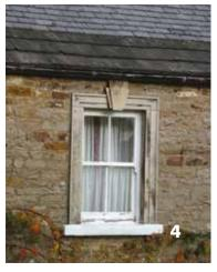
Close to these cottages is Moor View, also from the mid 18th century (photo 5) which also faces directly on to the road but has far less ornamentation. This two storey, three bay building is constructed of coursed sandstone rubble. The roof is pantiles with shaped kneelers and ashlar copings; the windows have raised ashlar surrounds and one over one sliding sashes; but the porch is a 20th century addition and appears a little out of place.
