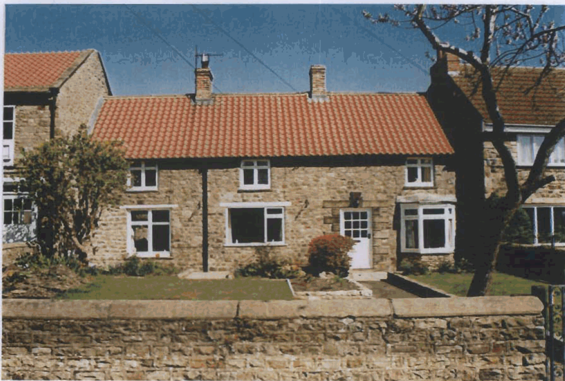
Ivy Cottage - traditional clay pantile roof. Note the imposing door casing with rusticated quoin surround and keystone
