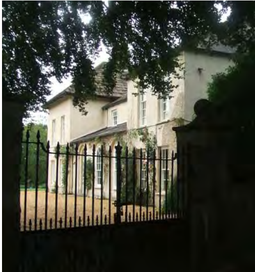
Grade II Listed Rectory, seen through its Grade II Listed gateway.
