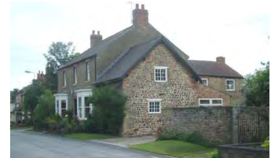
Grange Farm. The farmhouse is clad in roughcast, which was popular from the late nineteenth century onwards. The low gable and rear wing are faced with cobbles, typical of the way cobble was reserved for less prominent and lower status elevations and structures.
