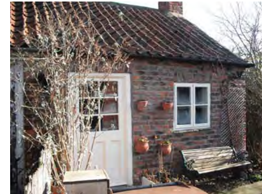
One of the two small cottages off Main Street formerly reserved for the poor and sick.
