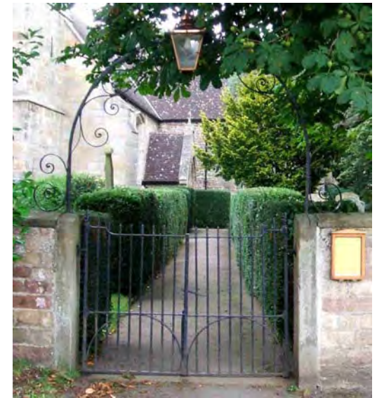
The listed iron gates and lantern overthrow at St Mary's Church.
