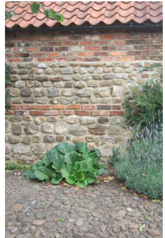
The use of traditional materials (in this case cobble walling, brick and pantiles) help this rebuilt building to complement its neighbours.
