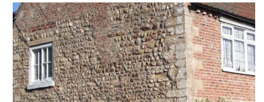
One of the few examples of stone quoins in Wath, and the only example of quoins separating brick to a front elevation and cobble to a gable.
