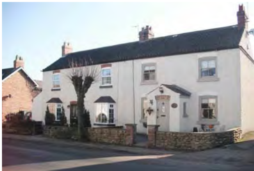
The regular spacing of openings gives this pair of vernacular cottages a more formal appearance than if the opening were offset from each other.
