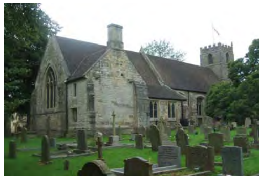
St Mary's Church. The gabled projection with the chimney is an unusual two storey vestry.
