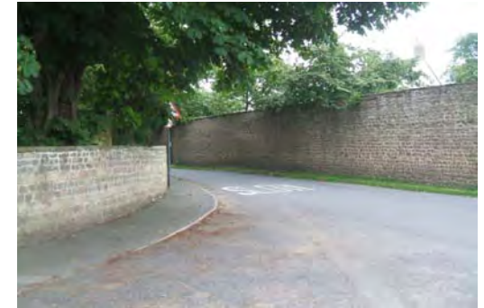
The cobble and rubble walls to the Church and Rectory are vital to the street scene of this end of the Conservation Area.
