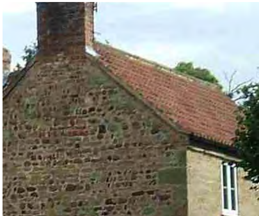
Stone was the highest status building materials in Wath (note the use of cobbles on the less important gable elevation).
