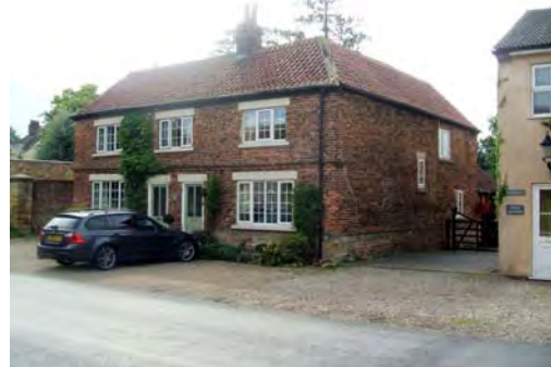
Church End. Note the stone and cobble plinth.
