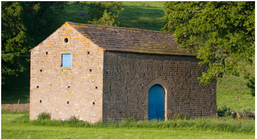
Above left: Stone slates. Above right: Typical Nidderdale barn with stone slate roof.
