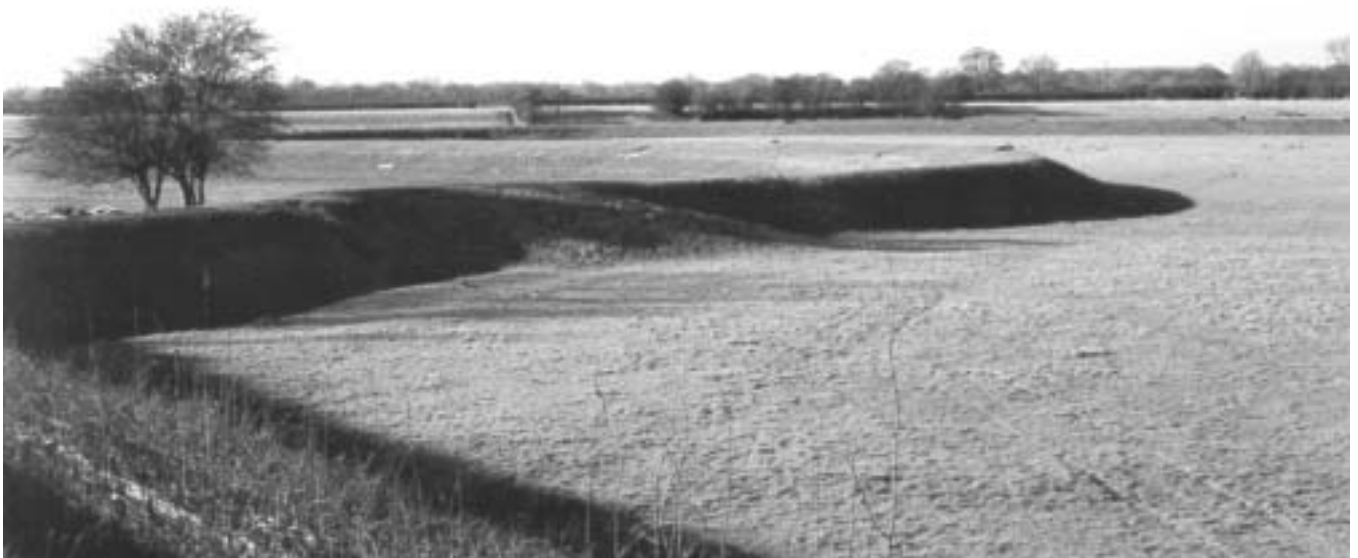
flood defences near Skip Bridge
