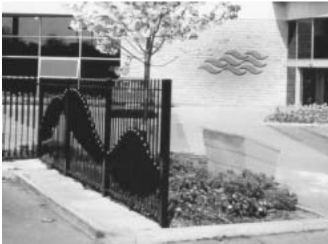
"Wave" fencing in the Hydro Swimming Pool car park continues the theme of the building's wave-like roof line and the facility's corporate logo.
