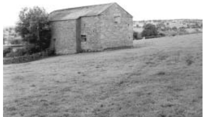
This barn sits comfortably in a wide open space and does not lend itself to conversion into a dwelling which would require the additional of a boundary wall.
