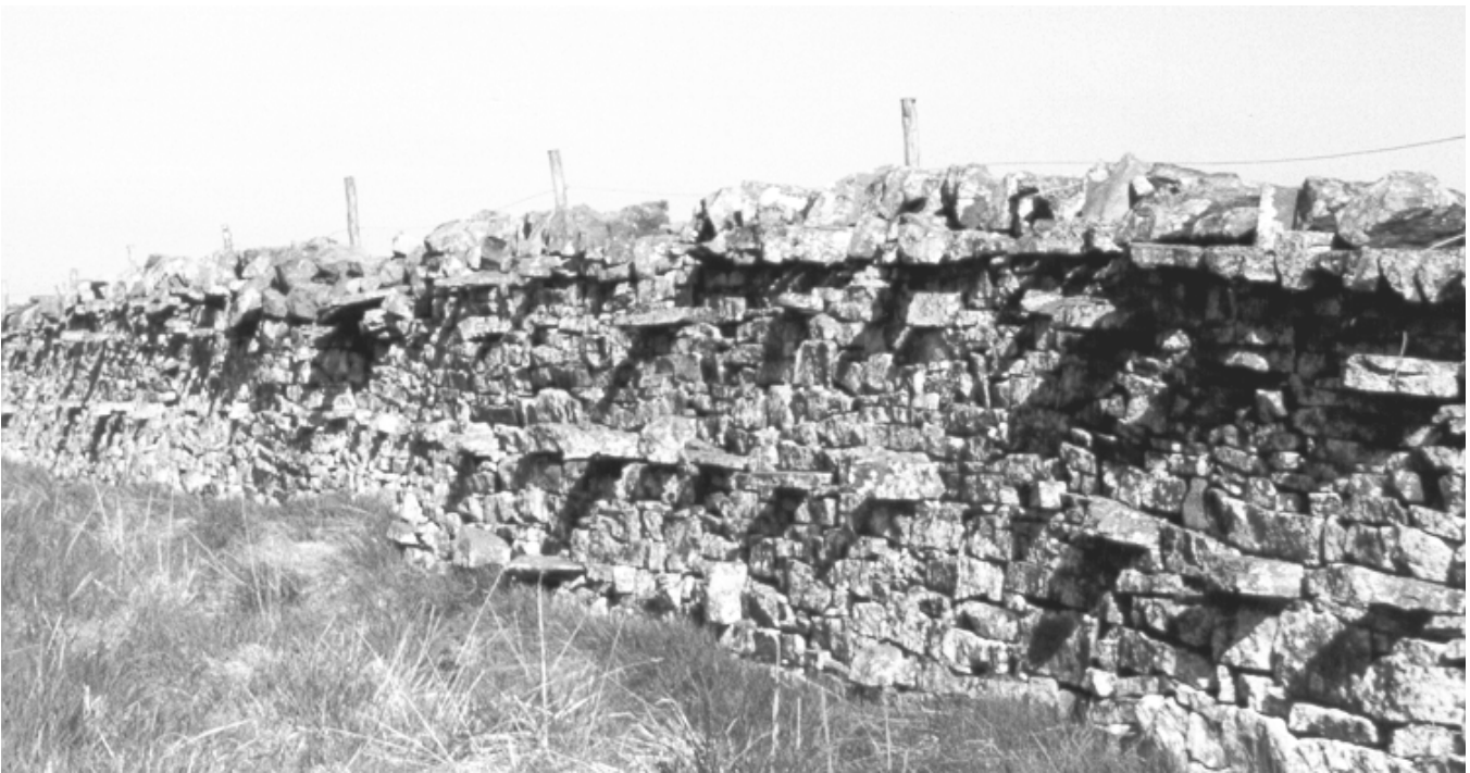
Masonry wall with square coping, Ripley Park.
