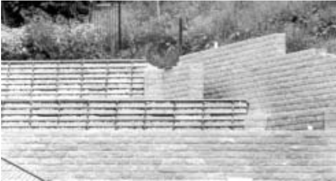
A crib-lock wall before planting up.
