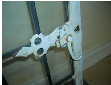
An example of a pre-19th century metal casement.
