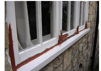
Just one example of a softwood window of no more than 25 years old showing severe signs of rot.
