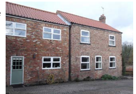
A poor example of an extension to a modestly scaled cottage – the extension is not subservient and the windows are poorly proportioned and out of character with the host building (which itself has suffered from the loss of its traditional sash windows).
