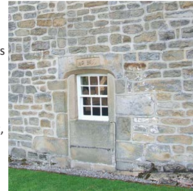
Although altered at a later date for another use, this historic doorway is still present and readable as such, thereby aiding the understanding of the building's history and also contributing to its character.
