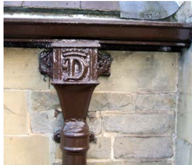
An example of traditional rainwater goods in Baldersby.
