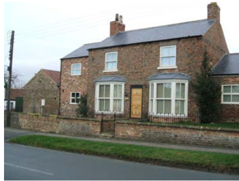
House extended both sides, both of different scale and subservient to the main block.
