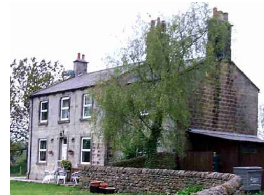
Cock Pit Farm. The regular spacing of tall openings on this vernacular buildings gives a well-proportioned 'no frills' version of the Classical architecture found in towns.
