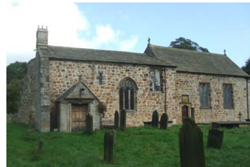
All Saints Church. Note the slender twelfth century lancet opening to the right of the porch, and the massive buttress to the left hand gable.
