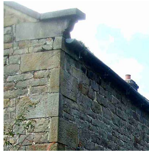
Quoins are found on both the vernacular buildings and the more architecturally stylized buildings in Weston.
