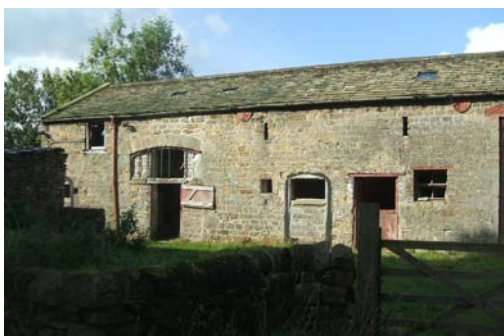
The barns at Cock Pit Farm
