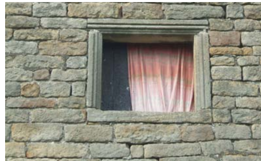
Gritstone. Although harder to work than sandstone, this rugged material was the most easily obtainable building material in Weston. The predominant use of sandstone in nearby Otley heightens the visual differences between these neighbouring settlements.
