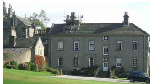
The western elevation of Weston Hall. The late Tudor north wing is the tall gabled structure on the left. The formal Classical western front dates from the early eighteenth century but conceals an earlier building.
