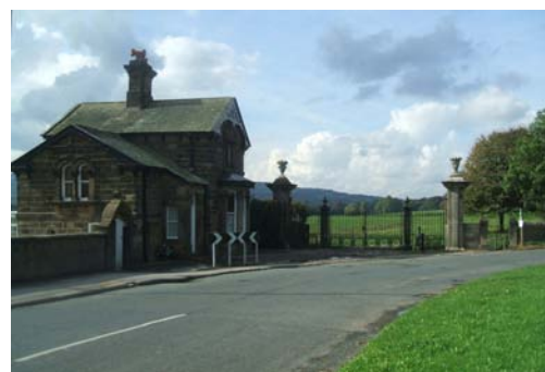
The east gate and lodge to Weston Park
