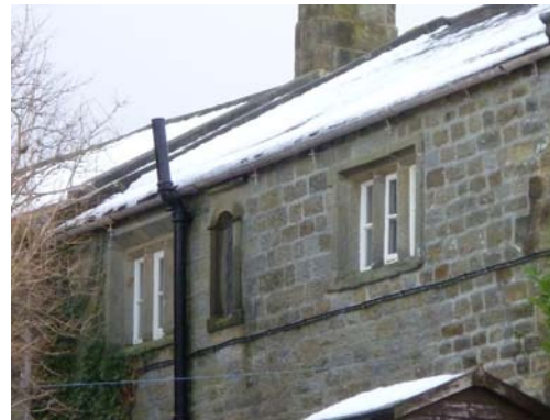
Details to rear of Woodman's Cottage, including mullioned windows.
