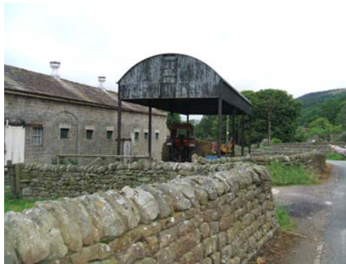
Contrasting farm buildings - barn dated 1861 behind a more modern Dutch barn.
