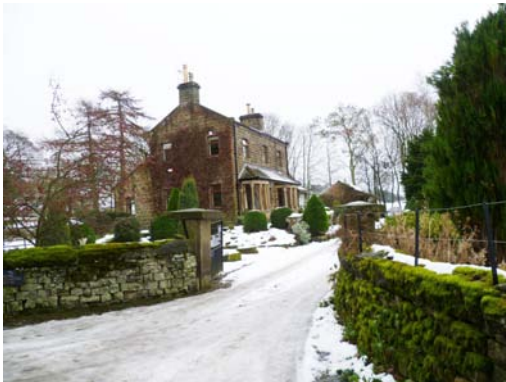
Rhyllstone House, the former Station building.
