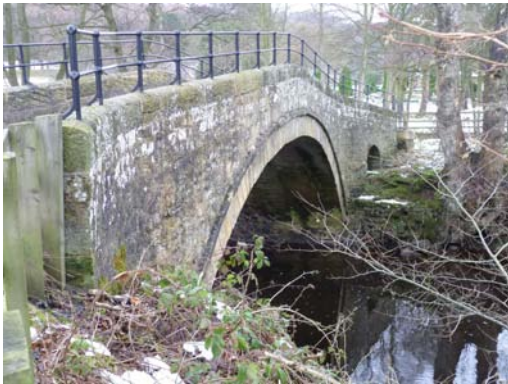
Wath Bridge (or ‘new’ bridge) altered in the nineteenth century.
