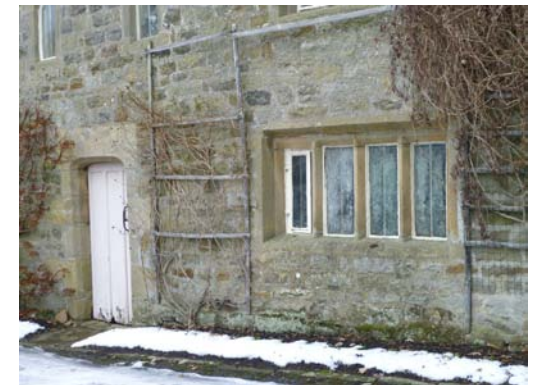
Detail of mullioned window and doorway at Sigsworth Cottage.
