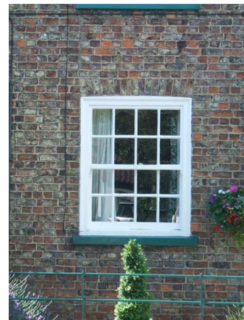
Small pane vertical sliding sash window.
