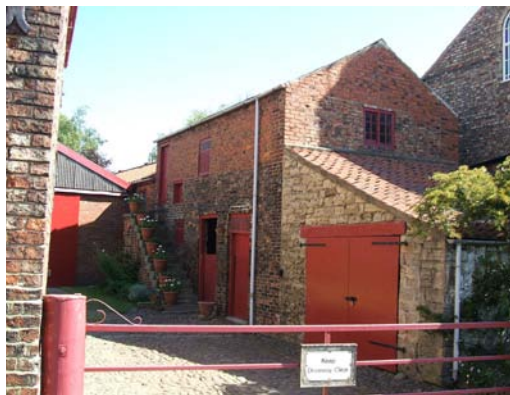
An old farmstead in a courtyard arrangement off the village street.
