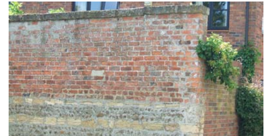
An important boundary wall now included in the Conservation Area.
