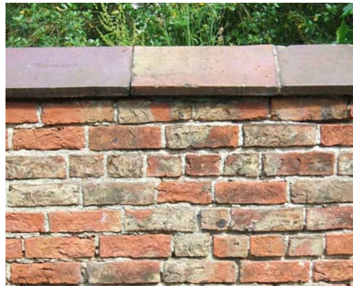
Brick wall with tile coping.
