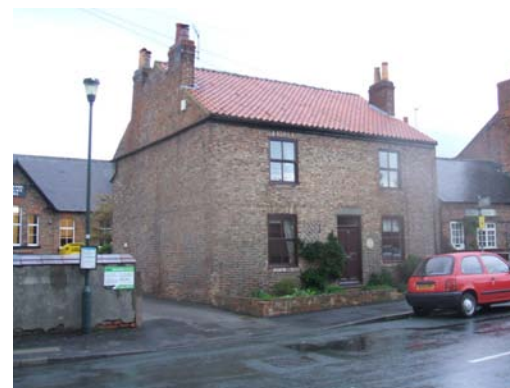
Chimney stacks with the thickness of the wall.
