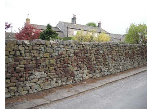
Stone paving against tall dry stone wall to the Garth.
