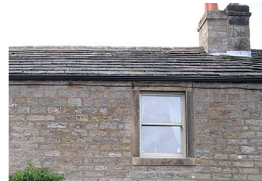
Vertical sliding sash window.
