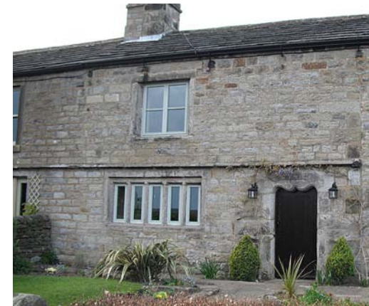
Casement window above mullioned window.
