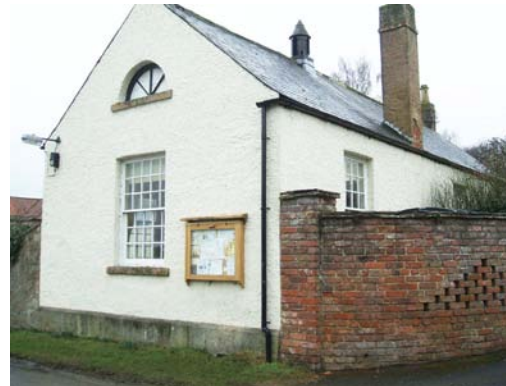
Village Hall roadside elevation.
