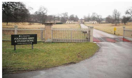
Piers and railings at driveway entrance to East Lodge.
