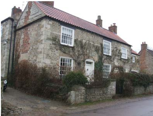
No. 25 Studley Lane is vernacular in style.
