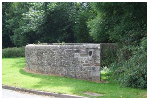
The walled pinfold enclosure, and the greenery around, it is a key feature of the Conservation Area
