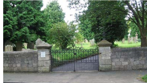
The principal entrance to All Saints' churchyard. These iron gates are dated 1897.
