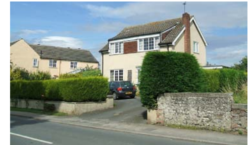
Moorfield. Ivy Cottage is to the left.
