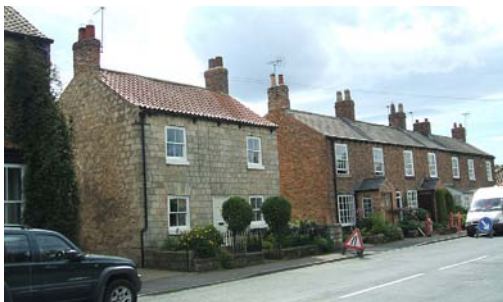
Traditional roofs and chimneys at Croft House and The Terrace
