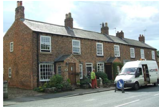
Local red-brown brick at The Terrace. Brick is the most common building material in the Conservation Area.
