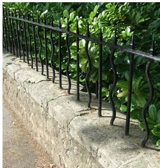
Cobble wall with stone copings and attractive railings at The Grange
