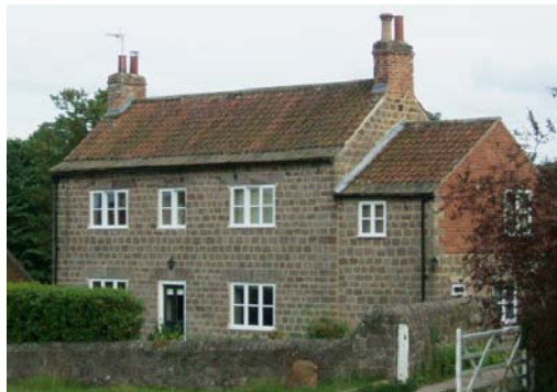
Oak Lea is built of most of the types of traditional materials found in Scriven.
