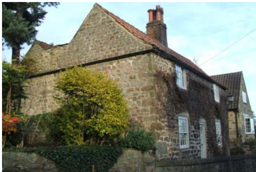
The Old Wheelwright's Cottage is made of traditional local materials. The twin gables indicate a double pile plan.
