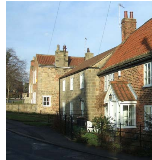
The Green's character is in part derived from the different types of buildings which face onto it.
