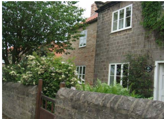
Sensitively designed extension at Spinney Croft.
