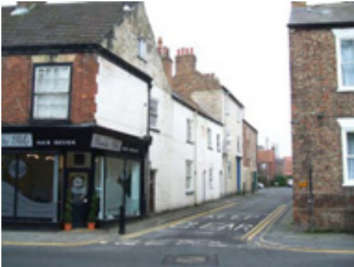
Re-fronting and rebuilding on King Street.
