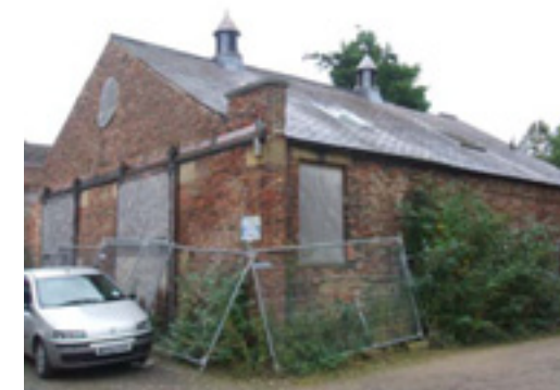
Rear of No. 40 Kirkgate
