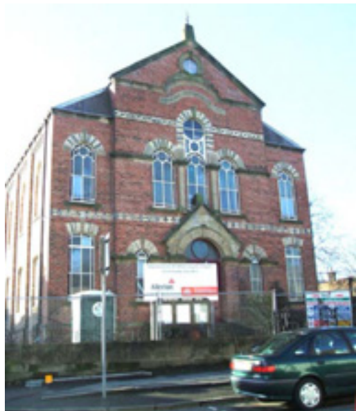
Former Methodist Church, Allhallowgate
