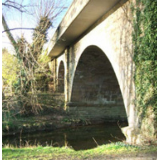
Skell Bridge, Ripon bypass.
