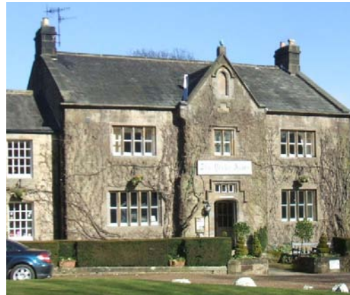
Stone mullioned windows.
