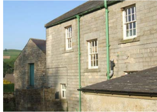
Vertical sliding sash.
