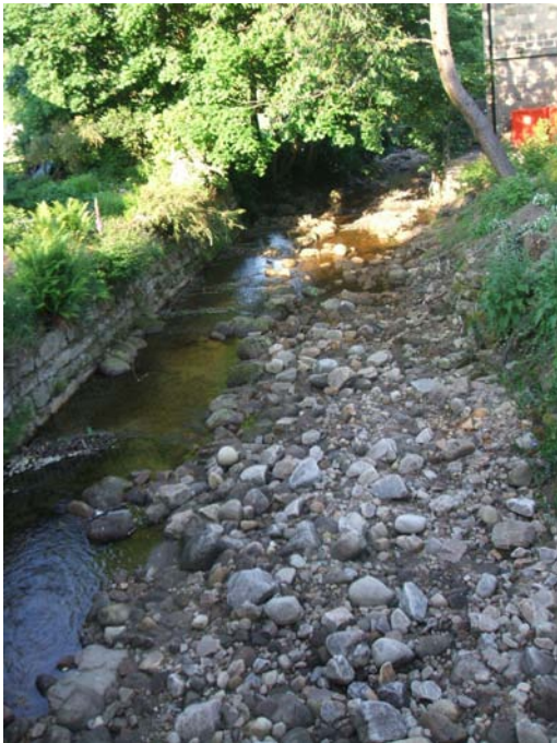
Beck showing low retaining wall to north side.
