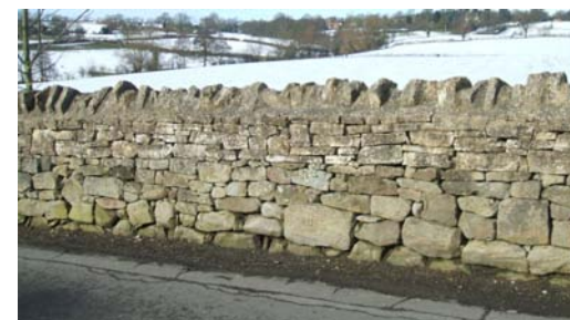
Wall opposite The Old School Room
