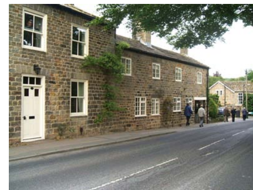
Nos. 12 and 14 Main Street, contrasting listed buildings
