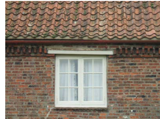
Paired casement windows and coggled eaves course.
