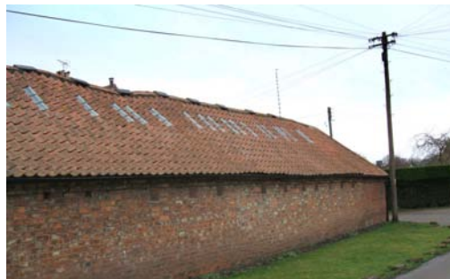
Overhead wires and telegraph poles are visually intrusive.
