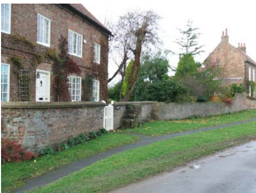
Front boundary walls are characteristic. Note the mounting block.
