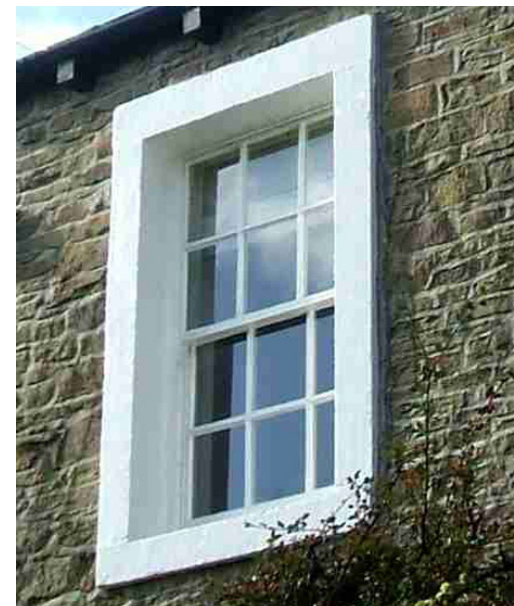
Projecting plain stone surrounds to a window opening.
