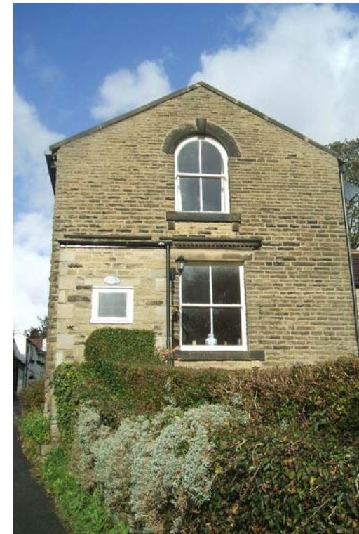
The gable end of Hawkesworth House.
