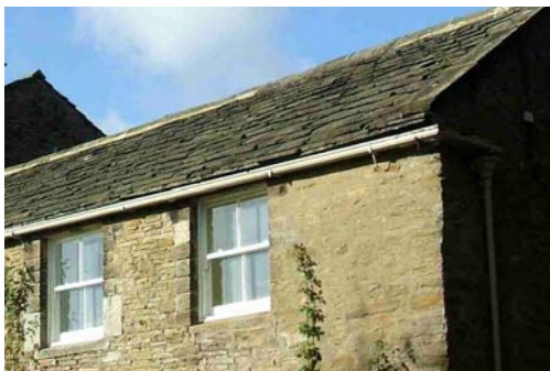
Plain eaves and tabled gables are typical features of buildings in Nesfield.
