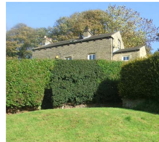
The buildings overlooking the ‘low green’ are perched above it.
