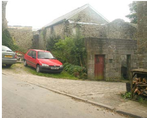
Building on the northwest corner of Church Farm.
