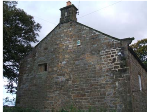
Traditional detailing, note chimney design, tabling terminated with kneeler and the quoin stones
