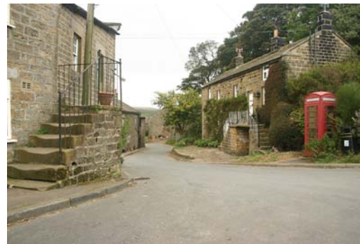
Blacksmiths Cottage (on the right).
