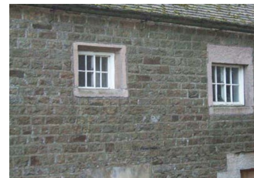
Yorkshire (horizontal) sliding sashes.
