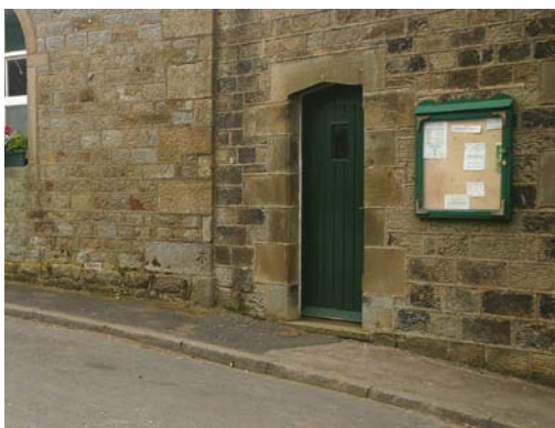
Quoins at the buildings' junction and on both sides of the door.
