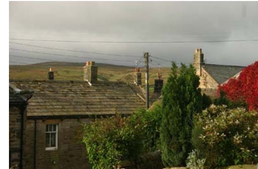
Stone slate roof
