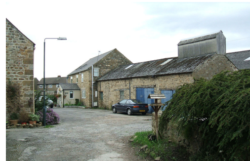
Quaker Terrace: a patchwork of development with housing and workshops
