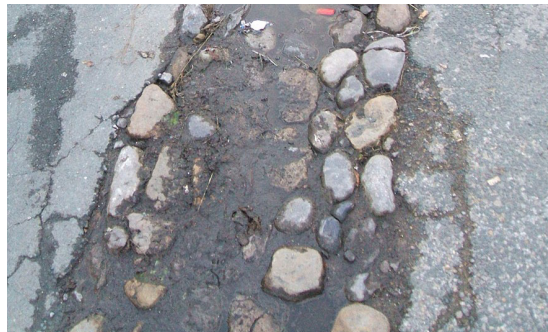
The distinctive cobble gully to the perimeter of the Market Place is being progressively eroded and would benefit from protection and enhancement. A level stone kerb to either side of the gully would provide a definitive 'stop' edge for the tarmac.
