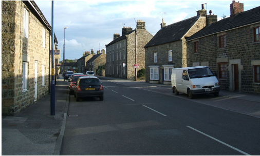
Properties 14-18 Park Street in the right hand foreground display a shallower pitch from the late-eighteenth century, while following building (No.24) clearly dates from the seventeenth century, both are of local stone with ashlar dressings and graduated stone slate roofs.
