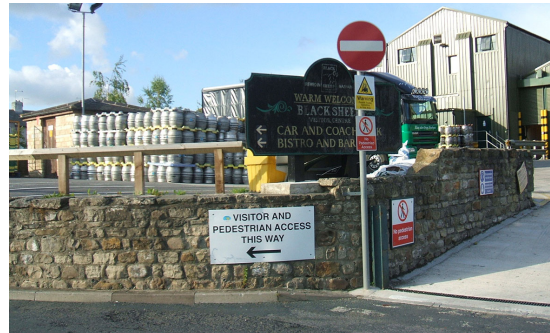
Black Sheep brewery – modern buildings outside the Conservation Area.
