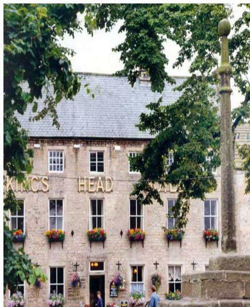
The Kings Head - eighteenth century former posting Inn and surprisingly Excise Office within the heart of the Market Place (Grade II listed). A coaching arch leads through to Kings Head Yard and open farmland beyond.
