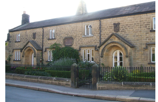
2-8 Swinton Terrace: the almshouses, although presently unlisted are without doubt 'landmark' buildings within Masham. Formalised front gardens and decorative railings demarking the boundaries are not common features in Masham.
