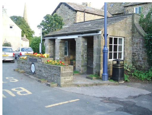
The southern side of Little Market Place is an untidy mix of the rears of properties, street furniture, shelters and hard landscaping.
