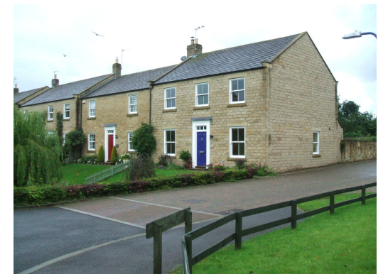
The western end of the Conservation Area is defined by new development around Swinburn Court. The general materials and details are sympathetic with Masham's vernacular and the open space in front is dictated by Swinney Beck which crosses in front of the properties (before eventually joining the River Burn).
