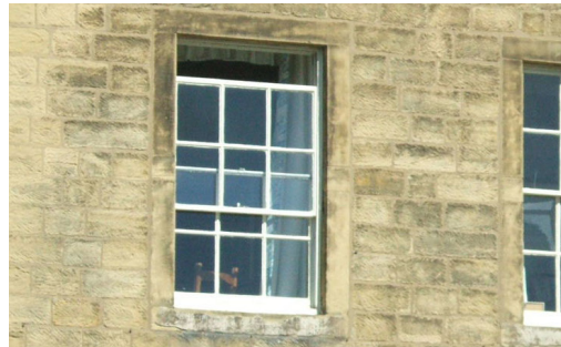
Vertical sliding sashes
