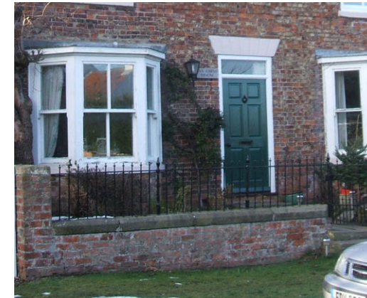
Panelled door with fanlight over.
