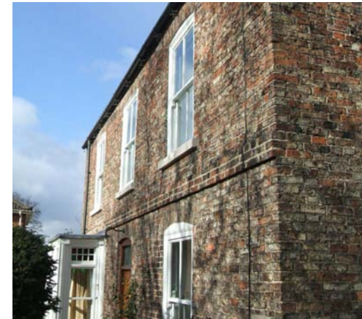
Brick walling with projecting floor band.
