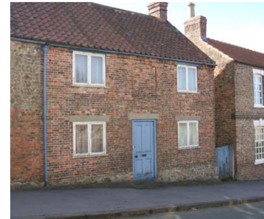
Simple four panelled cottage door (later concrete lintel).
