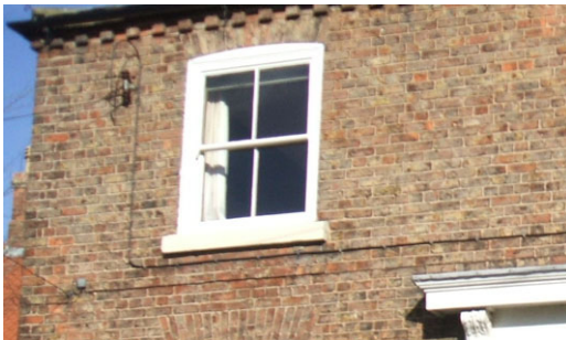
Stone cill, rubbed brick voussoirs and stepped and cogged eaves.
