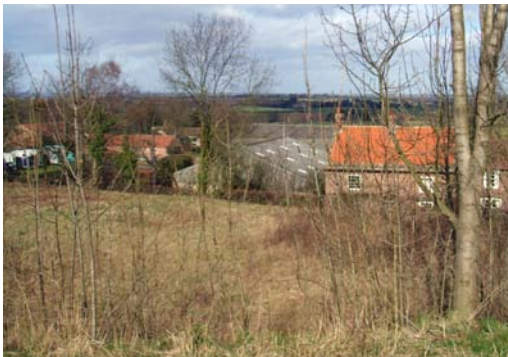
View across roofs of Prospect Farm.
