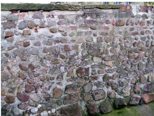
Cobble wall – small stones with shallow stone coping..
