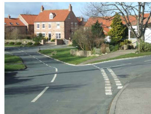
Redeveloped Town House Farm.
