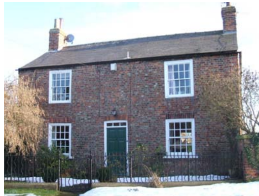
16 pane vertical sliding sash windows to house.
