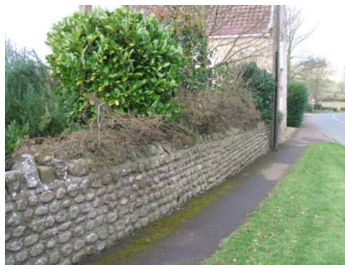
Cobble wall – larger stones laid to course with random coping stones.
