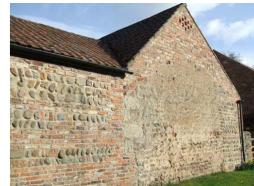
Outbuilding of brick and cobble with pantile roof.
