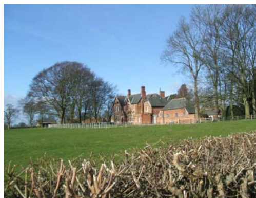
Marton Hall - former vicarage.
