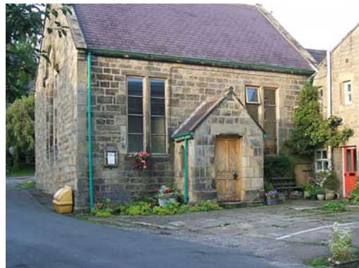
The tight stone flagged courtyard or square in front of the Methodist Church. Chapel Cottage is to the right.
