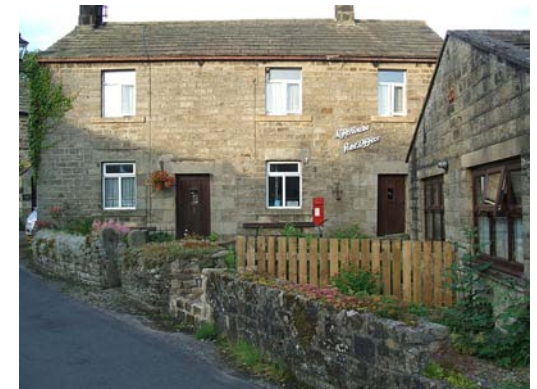
Lofthouse Post Office.
