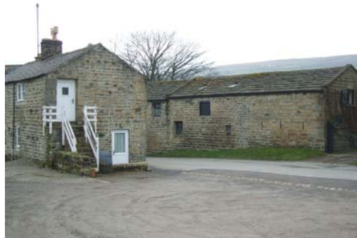
Holme Farm barn and Lund Cottage.
