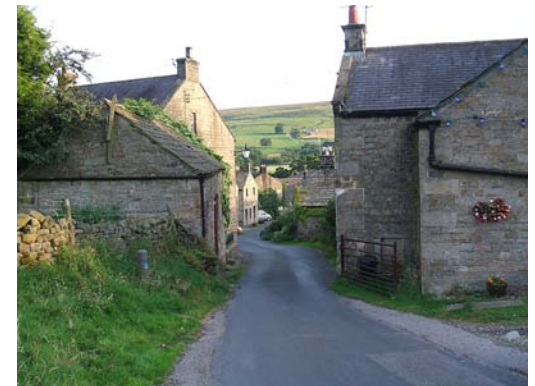
Entrance to village from Lofthouse Moor.
