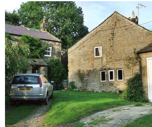
The asymmetrical gable of The Nook with The Cottage visible in the background.
