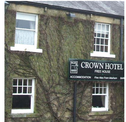
Sash windows through the ages: a Georgian-type sash (top right), a later Victorian sash (top left) and stylish Edwardian sashes (lower windows).
