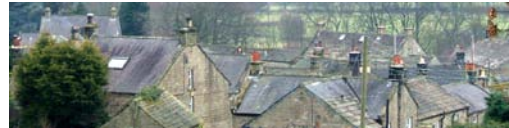
Roofs in Lofthouse are consistently ridged and gabled and retain traditional stone chimneys.
