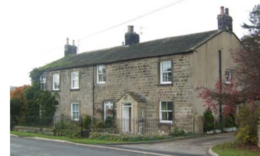
The retention of traditional sash windows has strengthened the group value of these three dwellings
