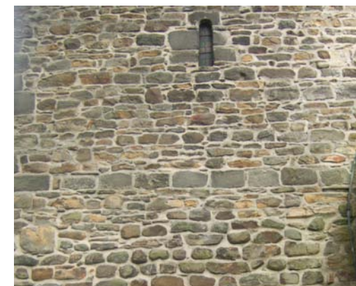
Coursed rubble with traditional lime mortar at St. Oswald's
