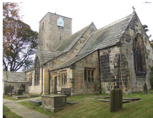
St Oswald's Church. Here we can see its Norman tower, and its extensively restored nave and southern aisle. The small mullioned windows and doorway may well be re-used parts of the 1470 re-build.
