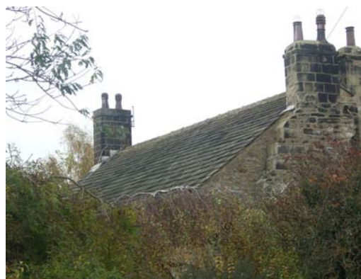
A typical roof in Leathley. The lateral stack on the right is not typical of the Conservation Area.
