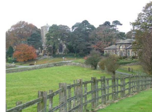
Almshouses & Village Hall across Park.
